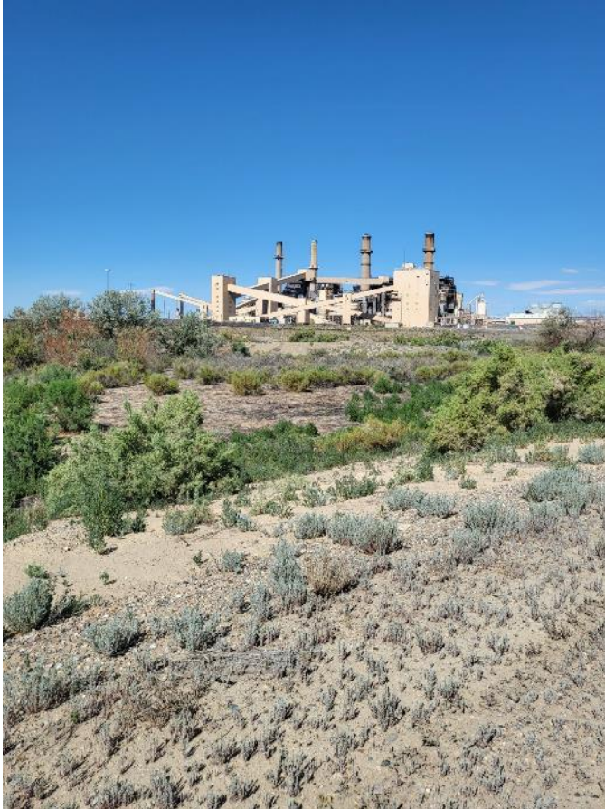
May 2023, prior to start of demolition
