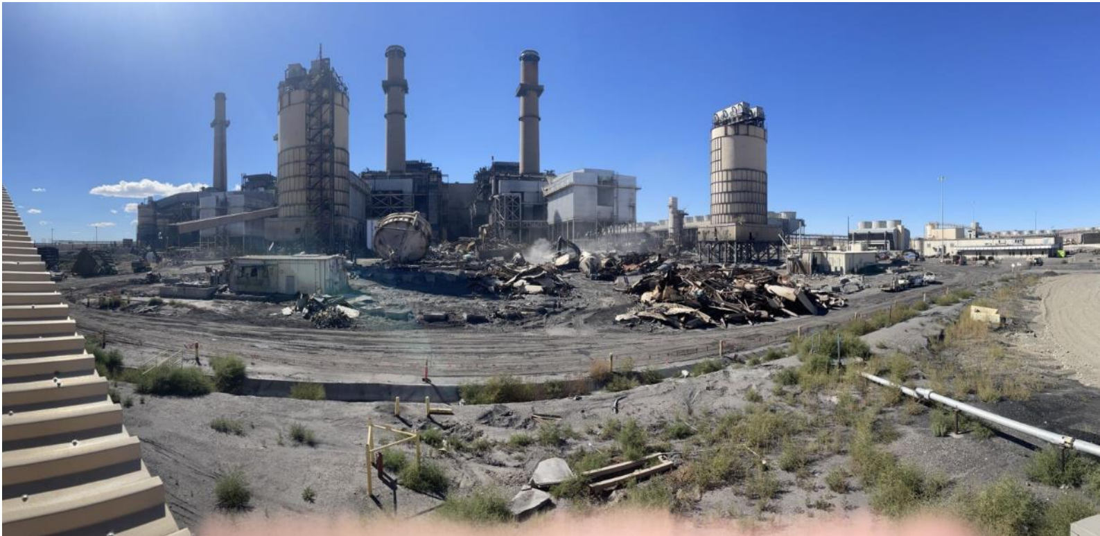
Wide Angle Showing Location of 3 Previous Pictures
