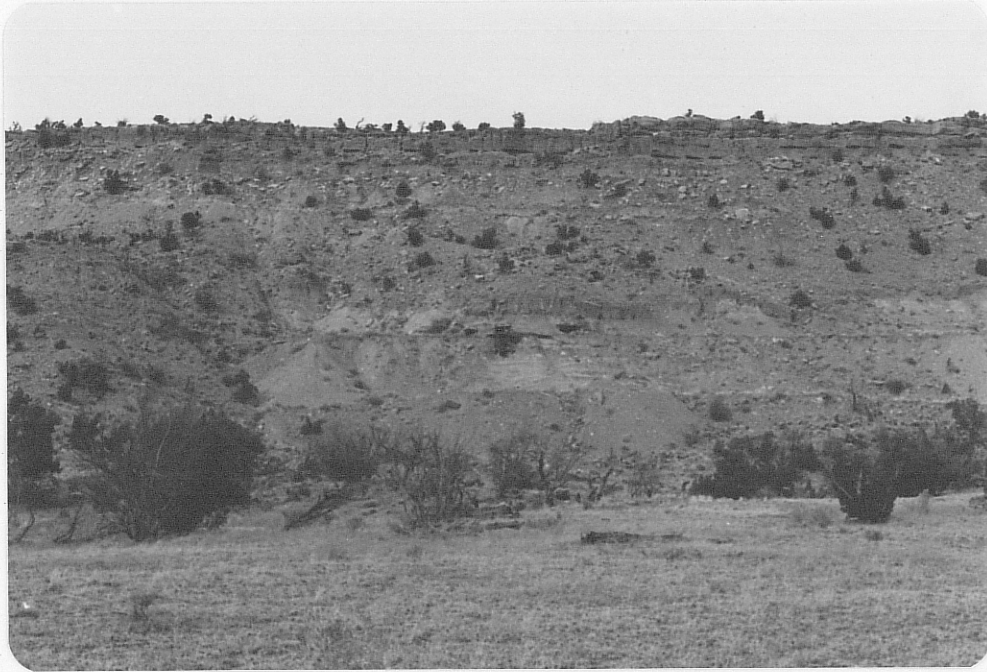
Photo (a) Looking northward at the Alta Mine showing upper face with adits, wooden ore chute (center) and lower loadout level.
