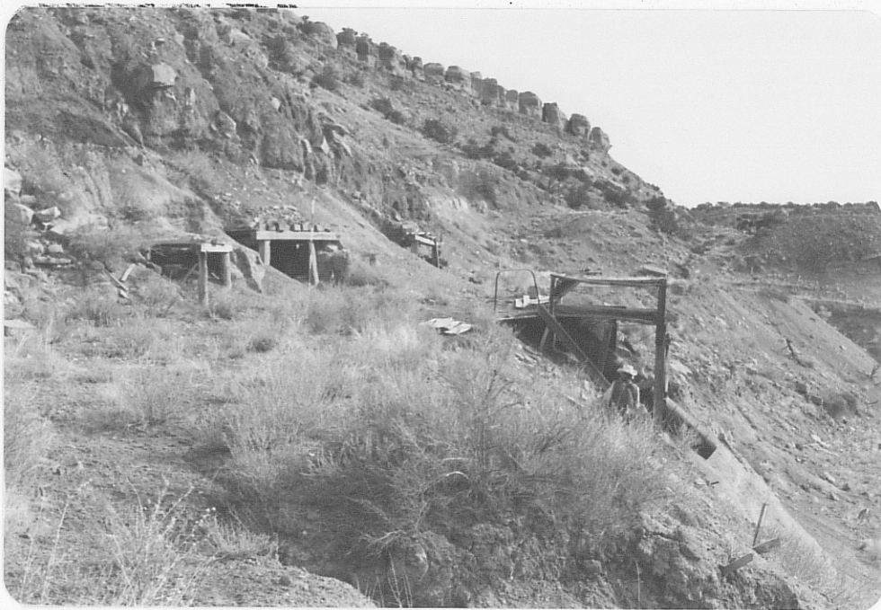
Photo (b) Looking eastward at the three adits driven in upper face and deteriorating wooden ore chute at right; note range pole at center adit for scale.
