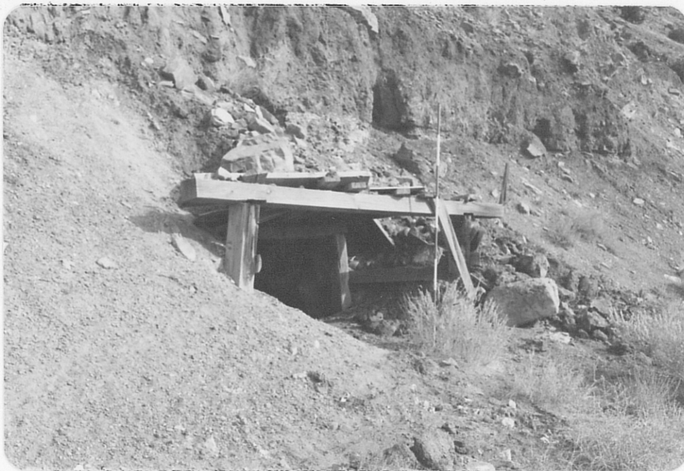
Photo (c) Looking northeastward at two adits at west edge of cut; adit at right behind range pole is main adit 50' or more in length.
