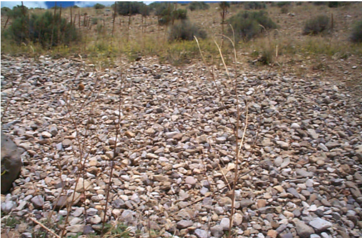
Photo 10: Close-up of the coarse rock layer at the toe of Dam 4.
