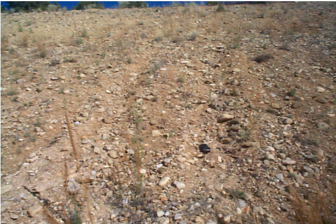
Photo 24: Moderate gullies in the east slope of the East Diversion Ditch at survey stop E-8.
