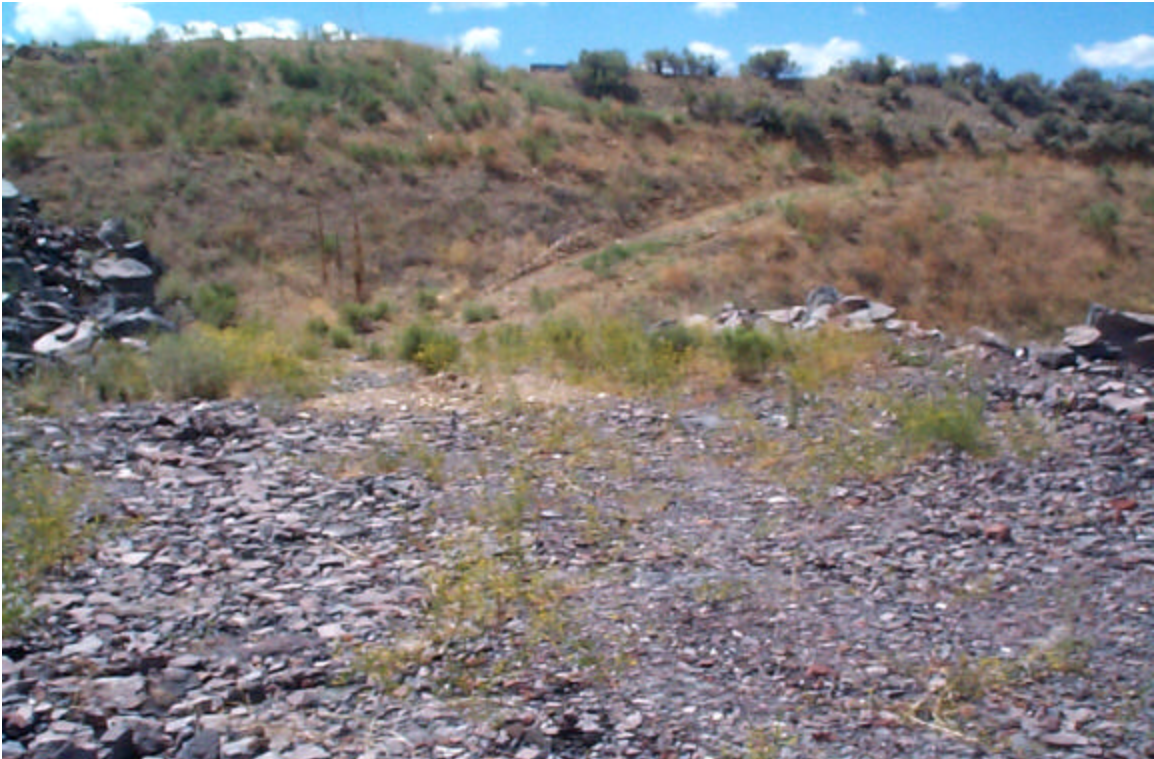
Photo 15: East abutment wall of Dam 5A.
