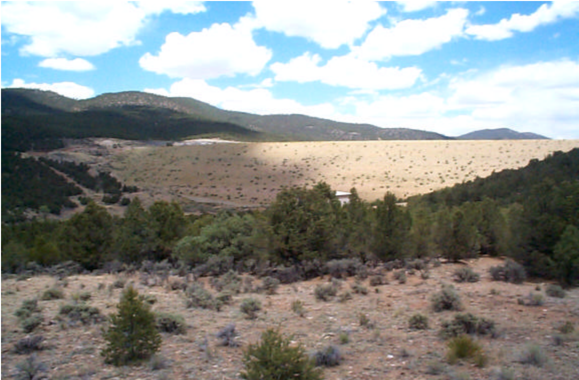
Photo 7: Looking north showing the downstream face of Dam 4.
