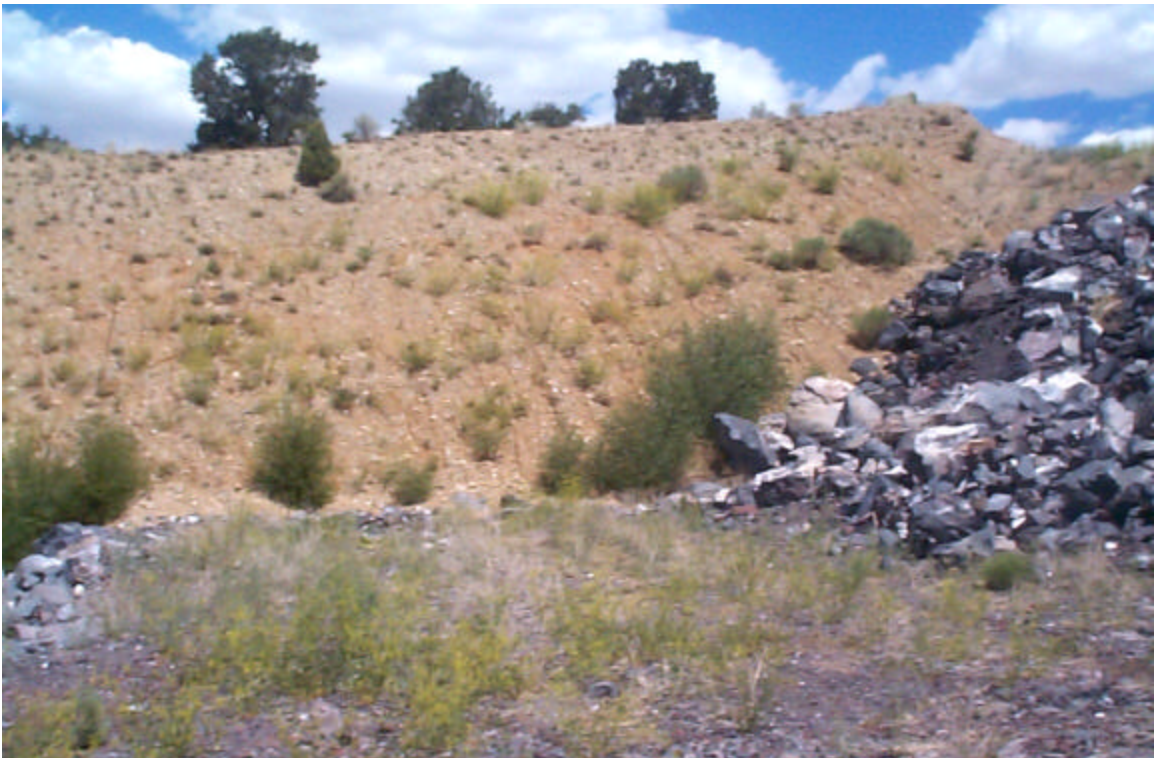
Photo 16: West abutment wall of Dam 5A.
