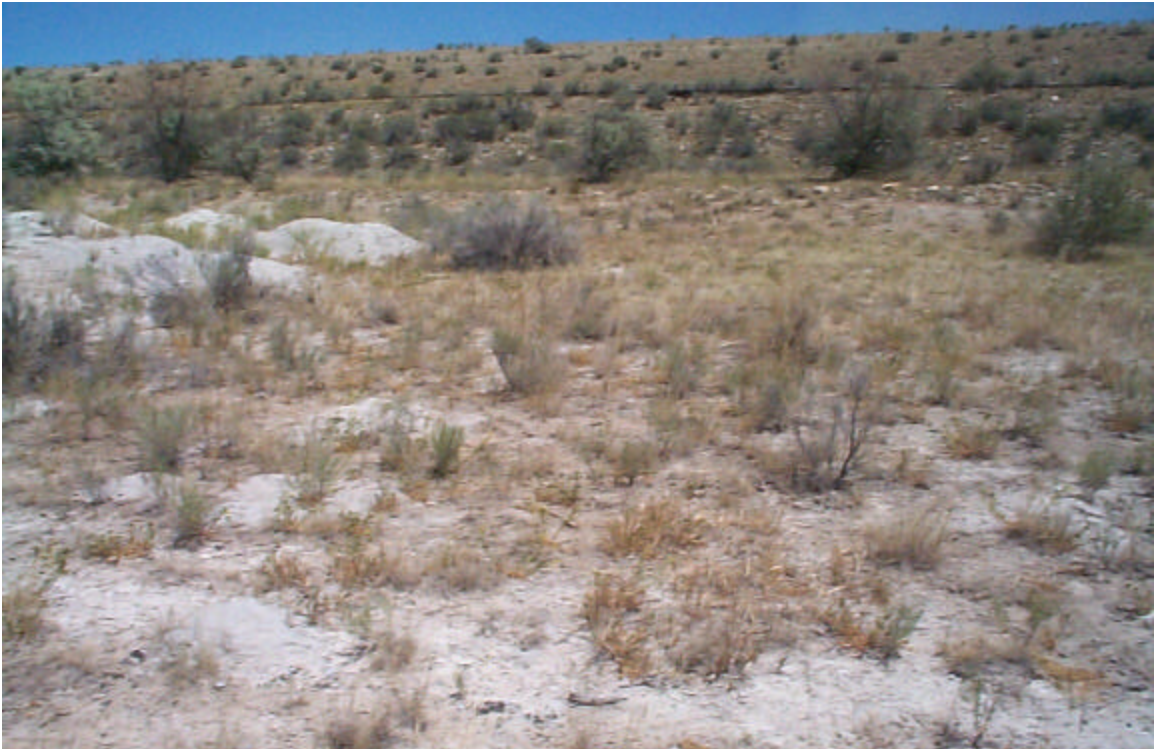
Photo 33: Tailings on top of interim cover material near the toe of Dam 1C.
