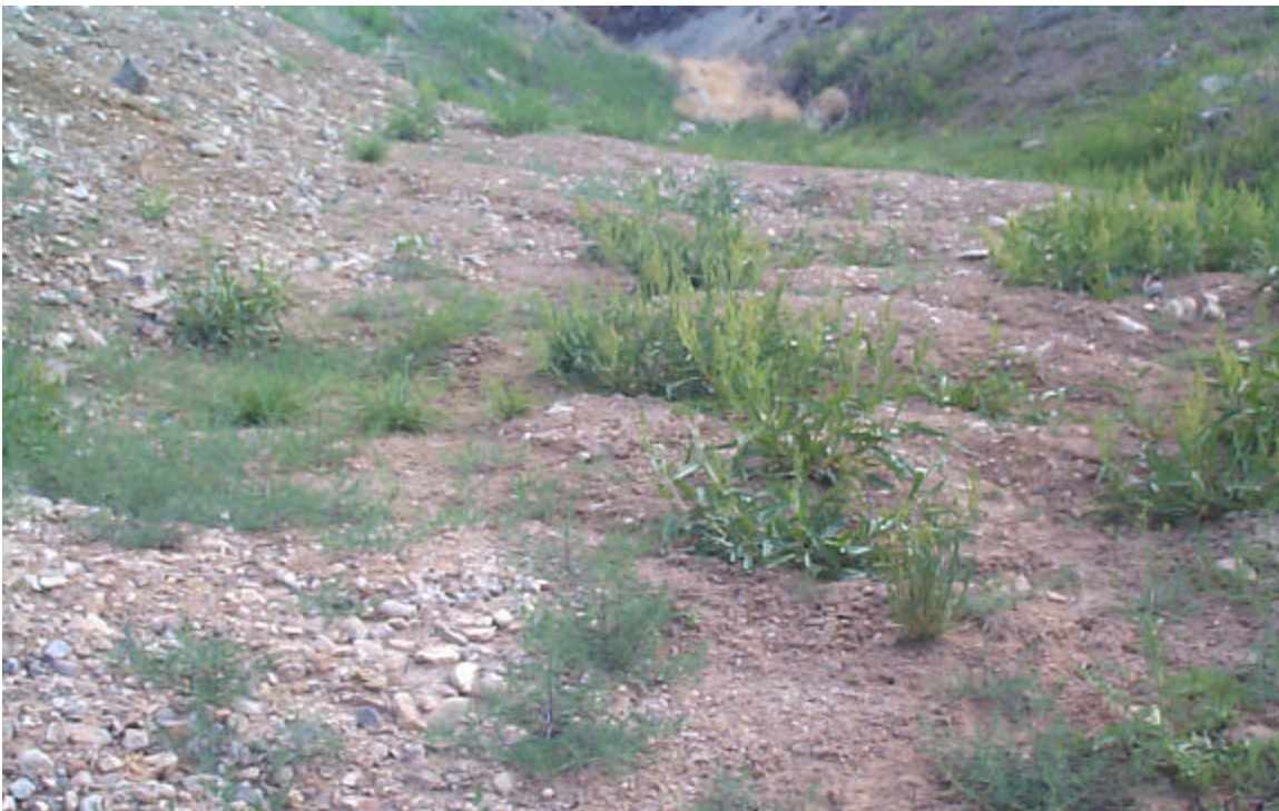
Photo 30: Earth flows originating from gullies in the east slope of the West Diversion Ditch at survey stop D-4.
