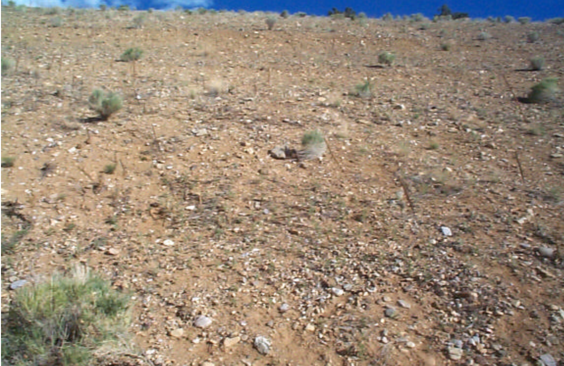
Photo 25: East/south slope of the East Diversion Ditch at survey stop E-10 (no erosion).
