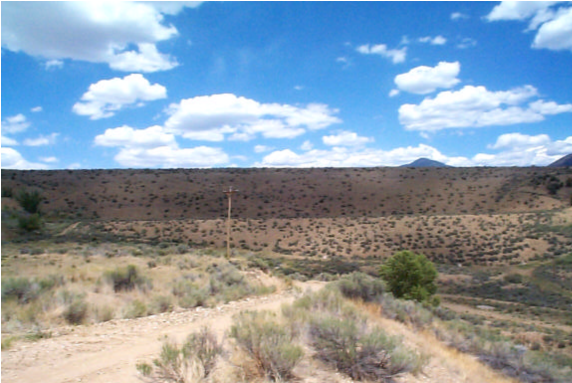
Photo 1: Looking north showing the downstream face of Dam 1.
