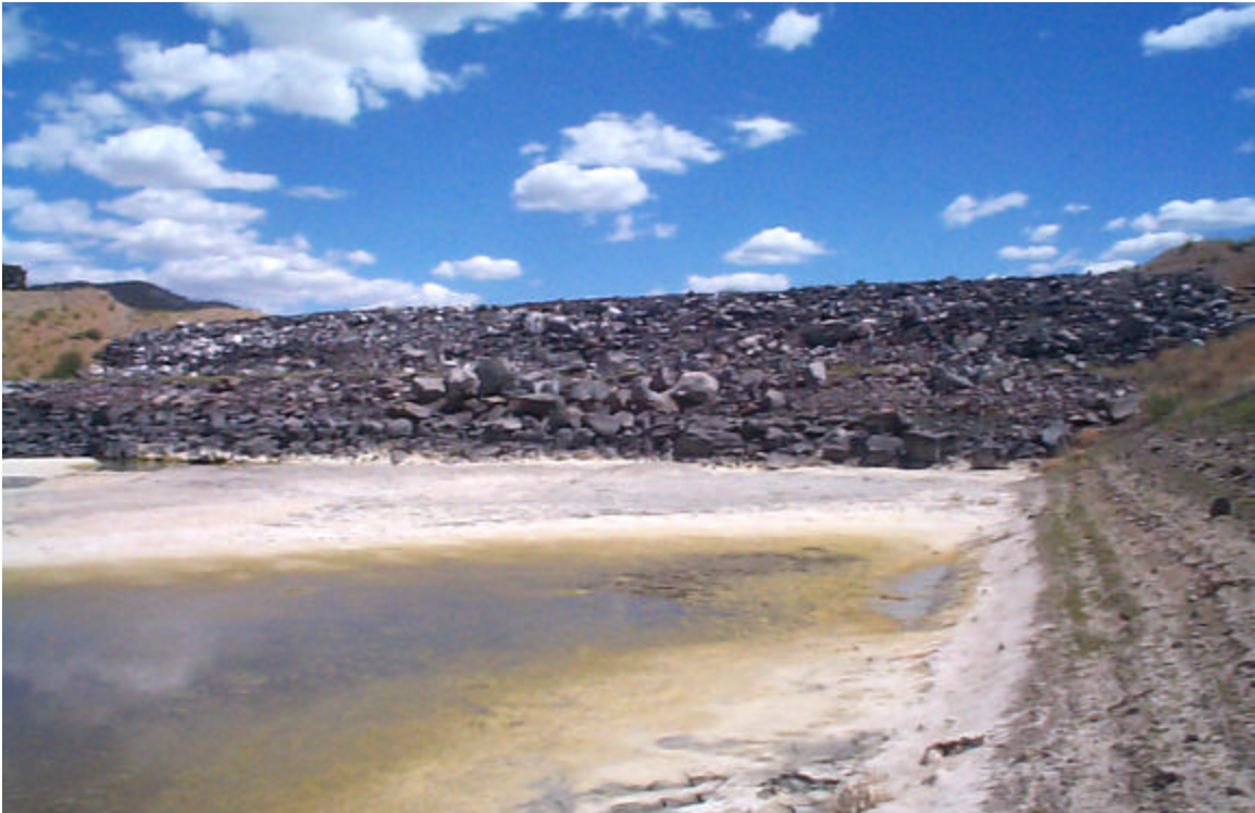
Photo 14: Looking north showing the downstream face of Dam 5A.
