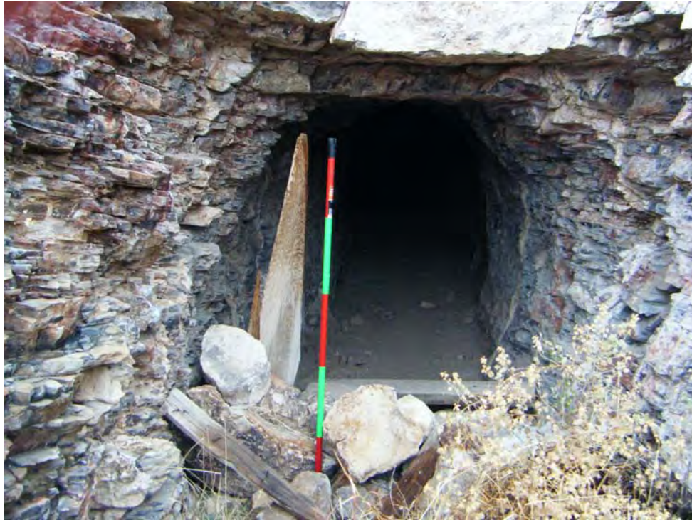
Photo 34-Looking west at Adit-2.
