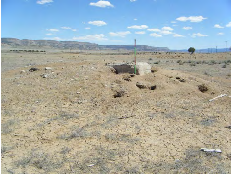
Photo 11-Looking east at PilePly-3.
