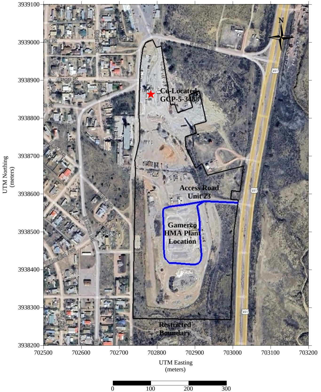
Figure 8-1: C&E Concrete's Gamerco HMA Aerial View showing Facility Layout
