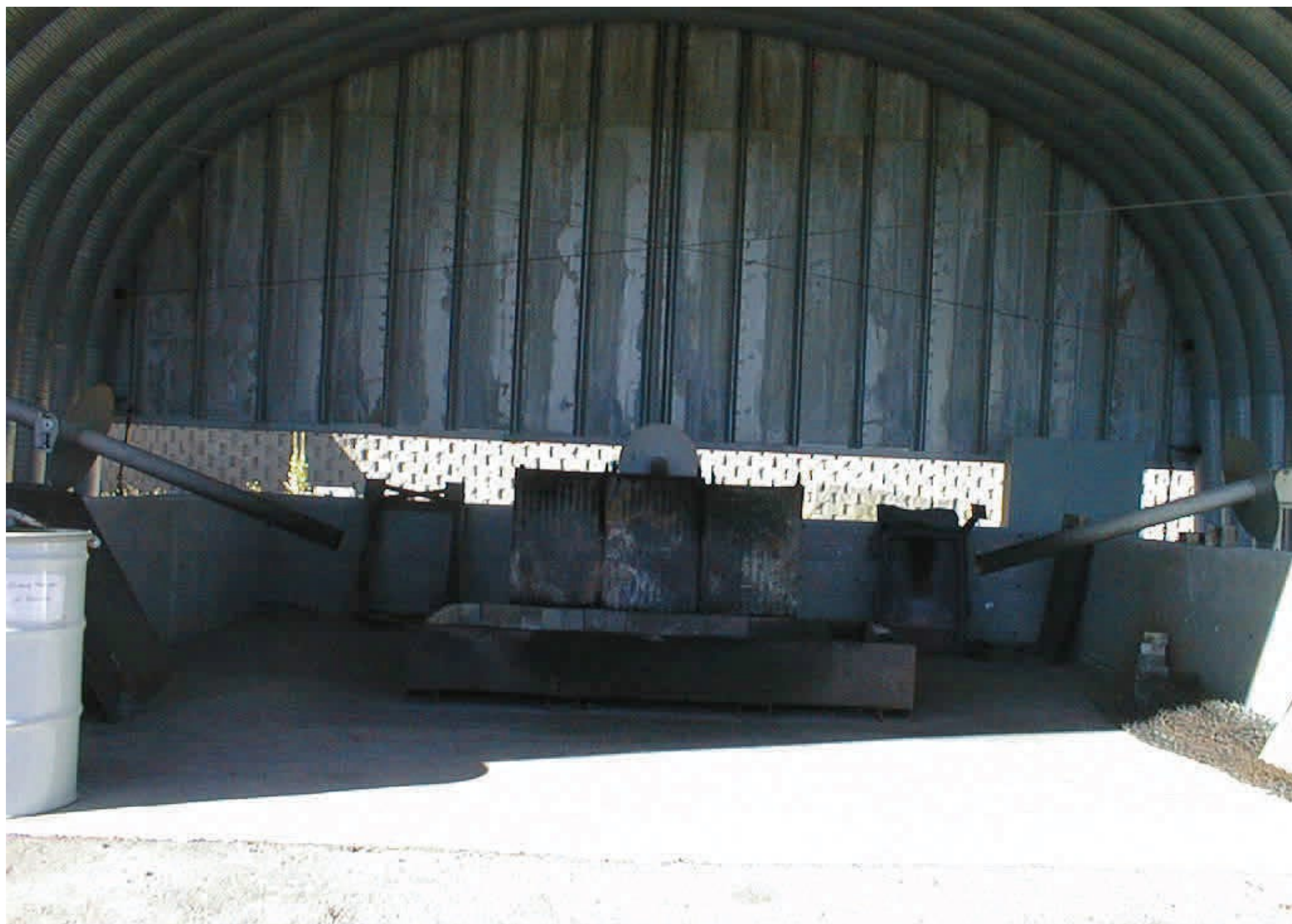
TA-16-388 Flash Pad Unit covered
