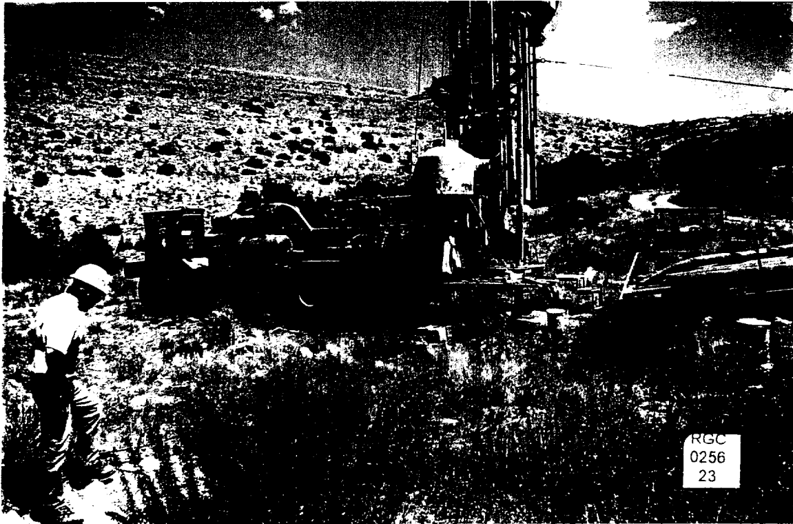
Photo 6: Drilling of monitoring well MW-13 at toe of Dam 4 looking northeast (photo taken August, 1997).
