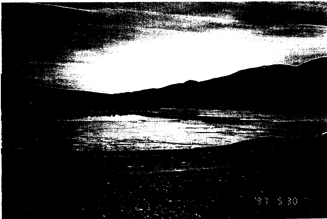
Photo 8: Tailings Discharge behind Dam 5A showing spigotted beaches and pond in background (photo taken May, 1997).
