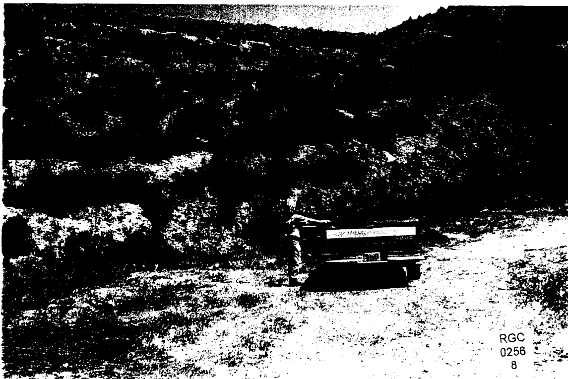
Photo 5: Toe buttress near east abutment of Dam 1 showing well-developed brush vegetation (photo taken August, 1997).
