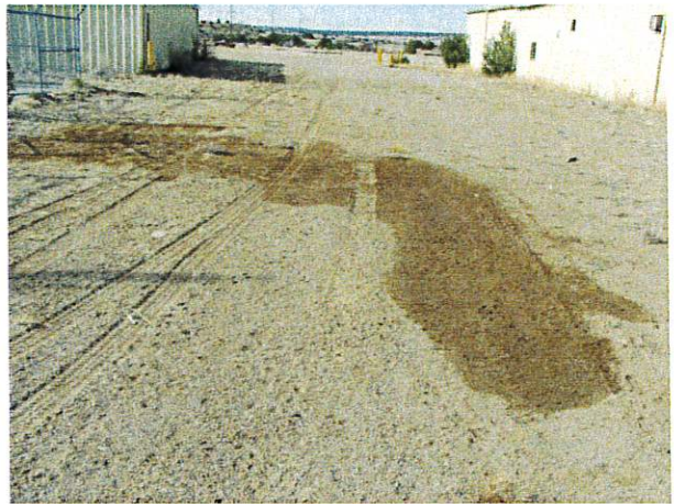
Transformer oil spill, recent tire tracks
