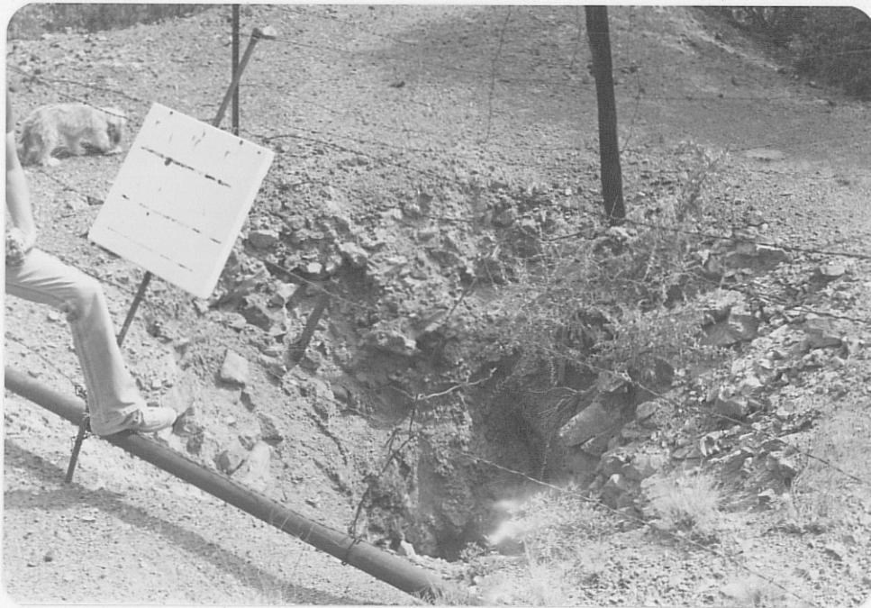
Photo (a) Merry Widow Mine shaft; 6' x 6' shaft is open down to about 40'. Fence is deteriorating but still effective. Sign is no longer legible.
