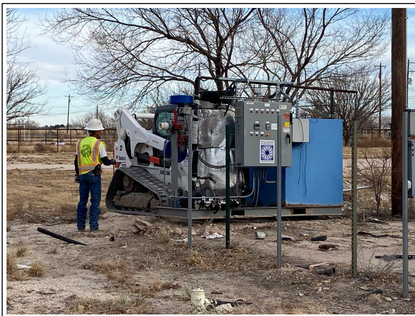
4. SVE blower skid during disassembly
