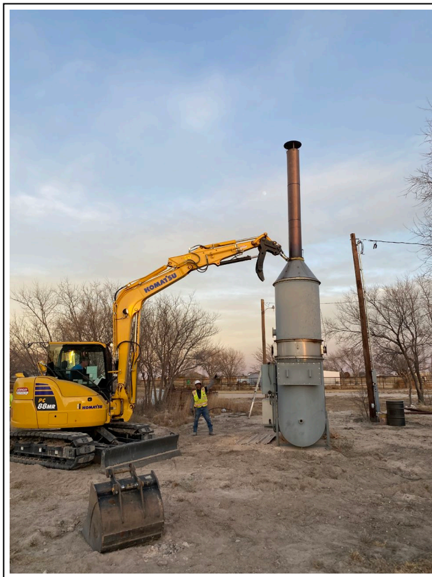
3. Oxidizer stack being removed at Lil's site
