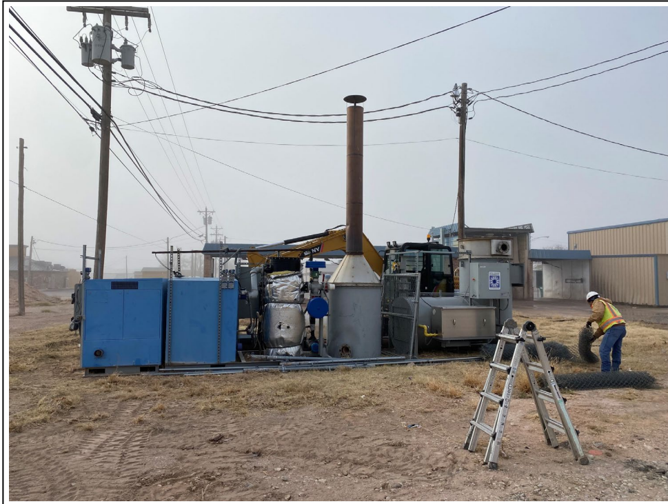
9. Oxidizer and SVE blower skid at Lovington yard after transfer
