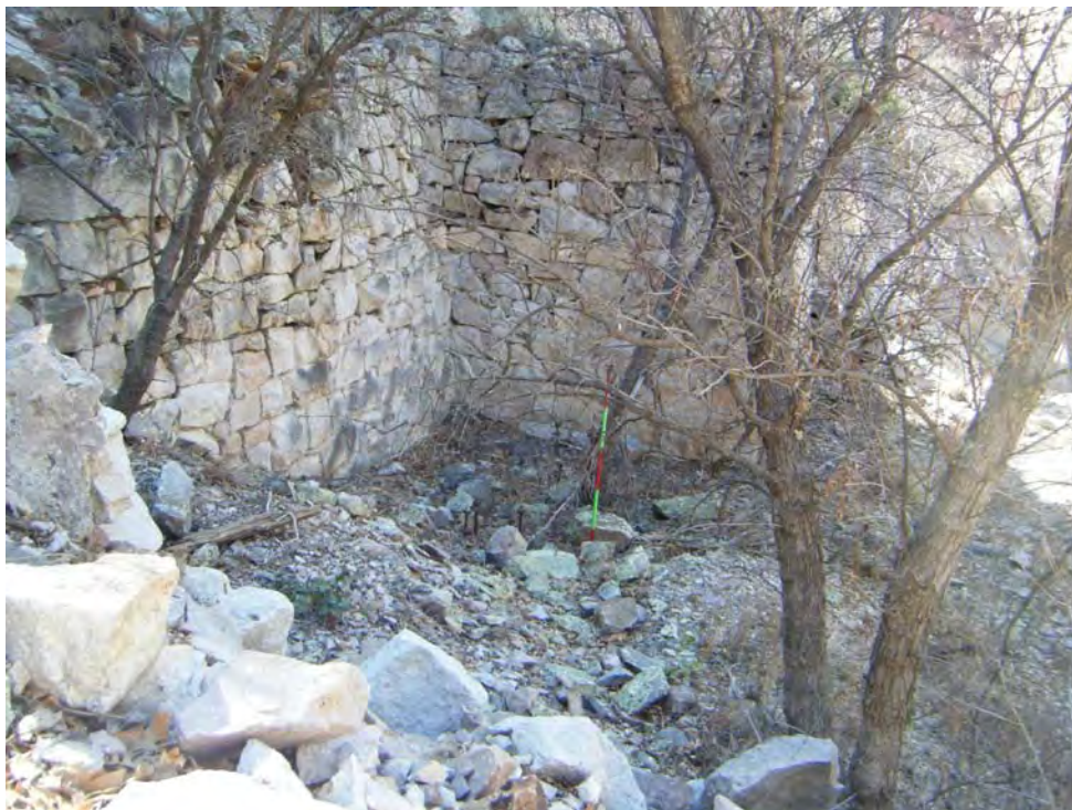
Photo 8-Looking west at LoadPly-1 located in the Eastern Area.
