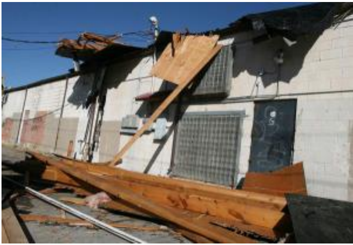
Wind gusts around 50 mph damaged this building in El Paso on October 25. (Victor Calzada /El Paso Times)
