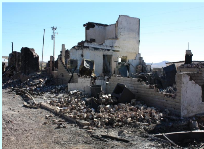
An electrical fire destroyed this building in Hueco Village TX after winds blew down nearby power lines. (Greg Lundeen NWS/NOAA)
