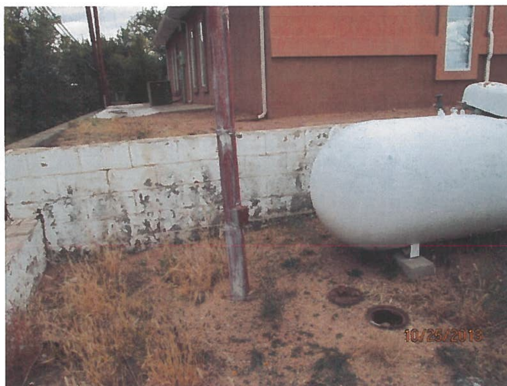
Photograph 4. View of MW-2A, showing location near propane tank near northwest corner of site building.
