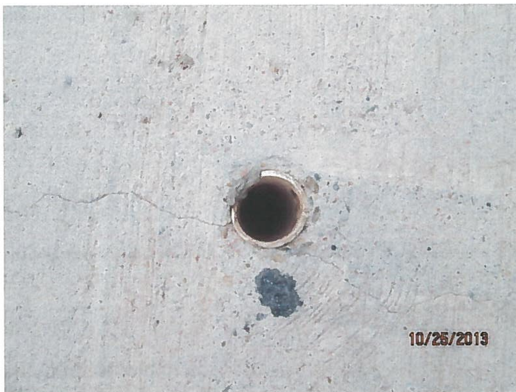
Photograph 1. View existing monitor well MW-1 in concrete slab pavement.
