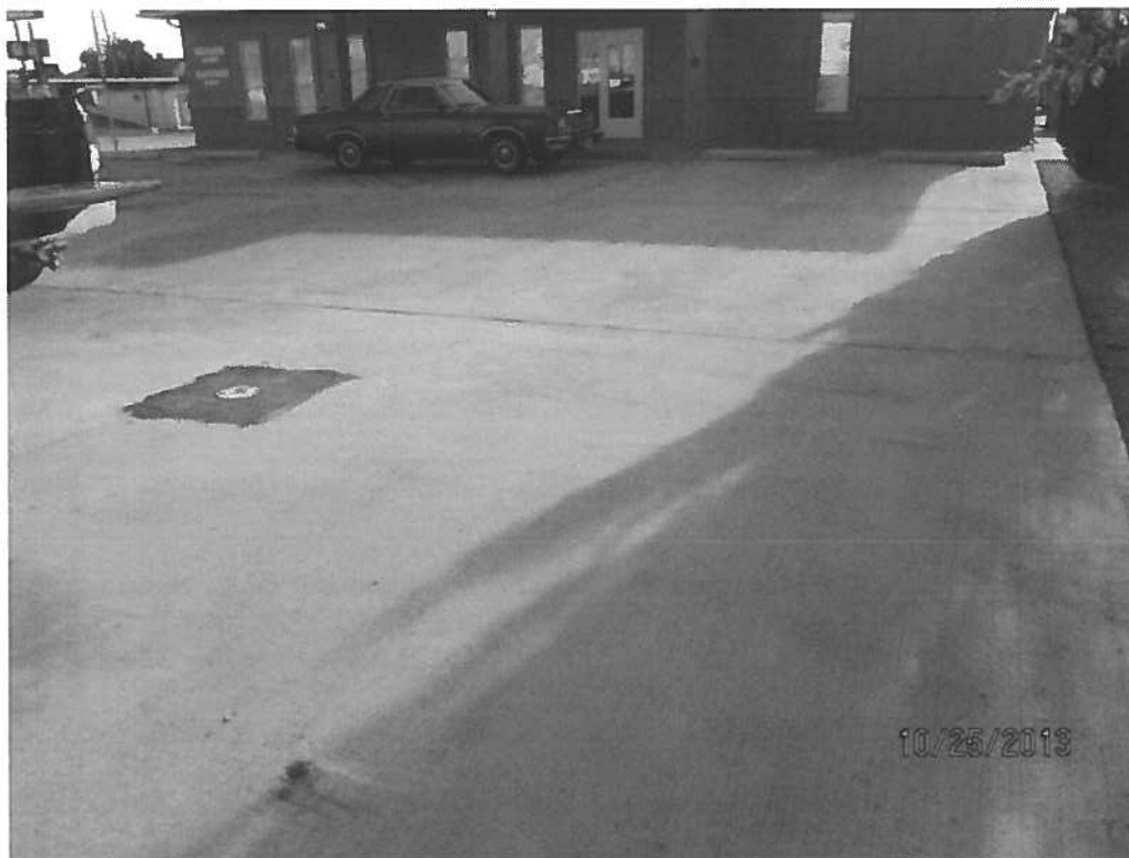
Photograph 8. MW-1 casing (lower left) and replacement well MW-1A located 9.9 feet away, looking toward site building.
