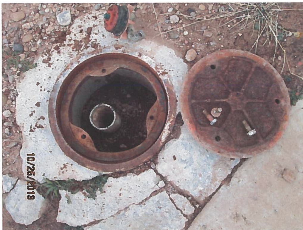
Photograph 5. MW-3 casing and well cover, with cracked concrete collar.
