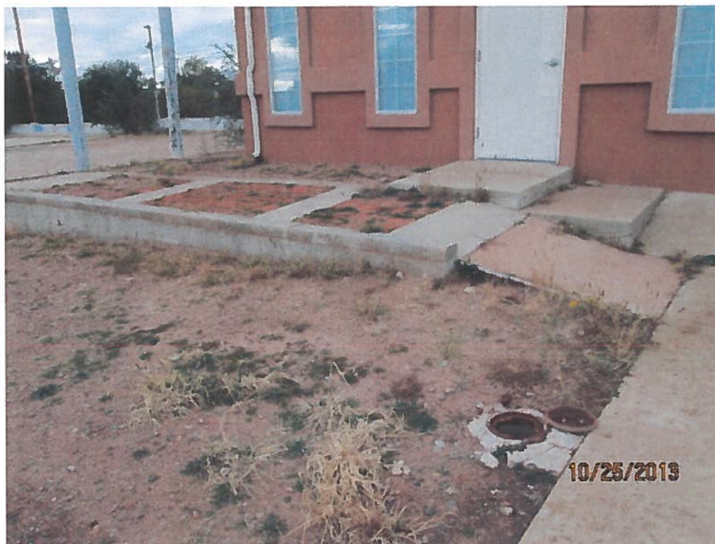
Photograph 6. View of MW-3, showing location near south-central side of site building.
