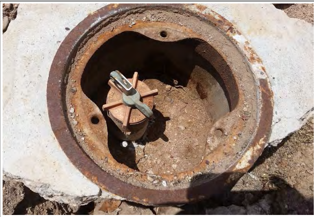
2. Interior of monitor well MW-3 well vault.
