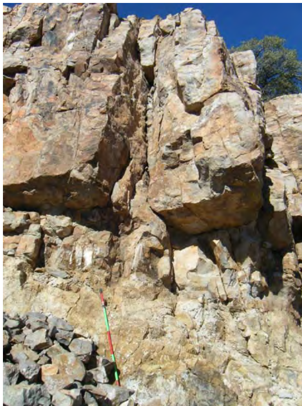
Photo 37-Looking north at the rock face of CutLn-2 located in the Southern Area.
