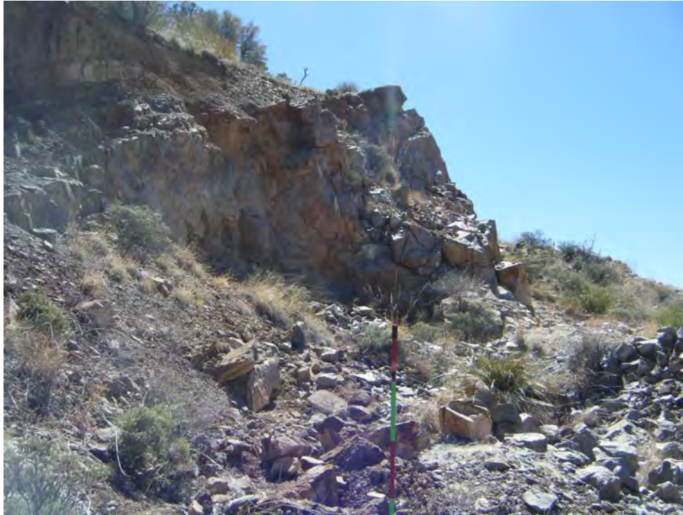
Photo 7- Looking south at an Open Cut (CutLn-1) located in the Southern Area.
