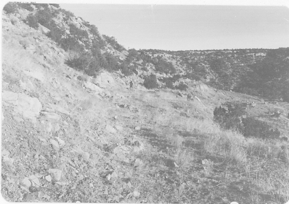
Photo (c) Looking E at 110' long bulldozer cut on Foutz 2 claim.
