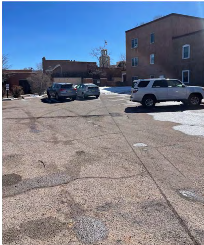
Cleaned up Surfaces before De-Mobilization
