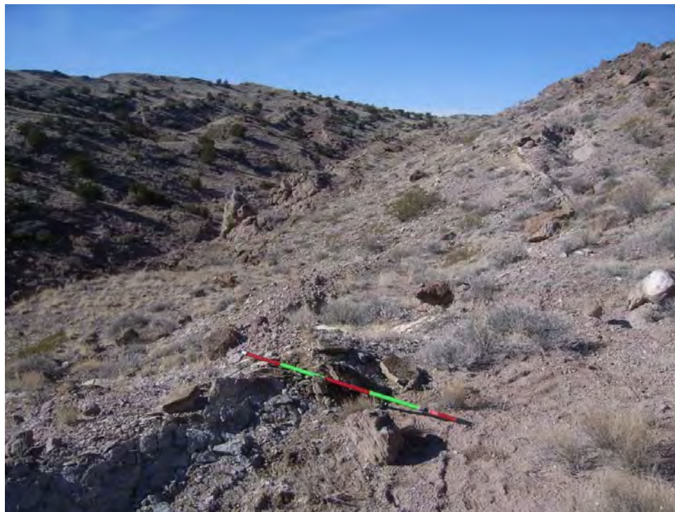
Photo 7 - A shallow cut (cut-1), possibly a bulldozer cut. The rocks scattered to the left of the scale pole have radioactivity readings of 240 \mu R/hr.
