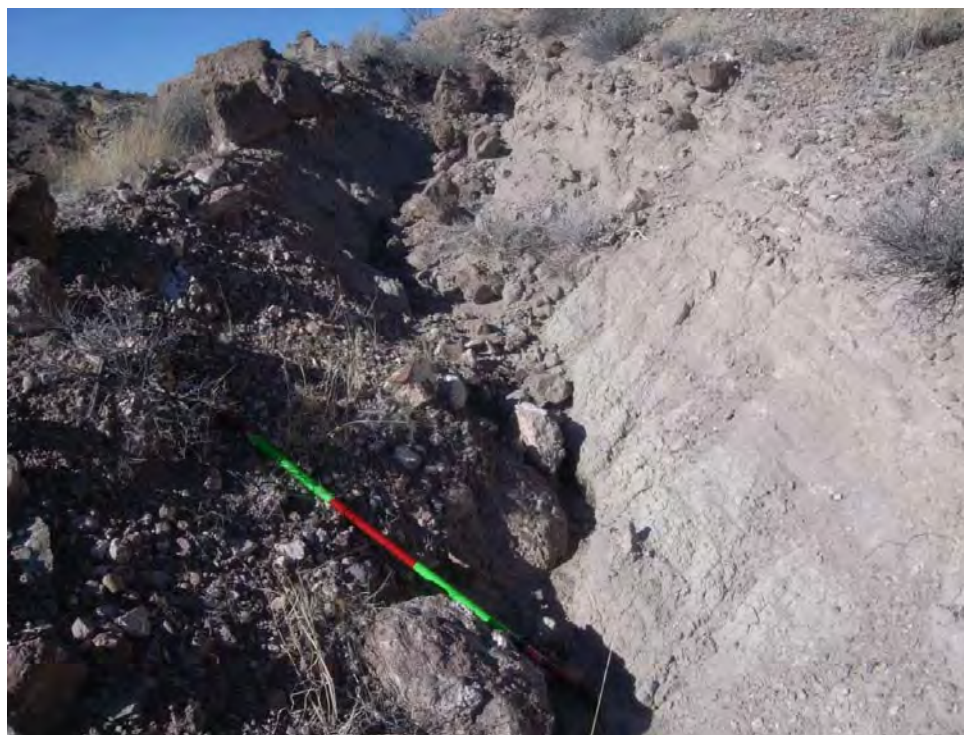
Photo 8 - A shallow cut (cut-2), possibly from a bulldozer, appears to have been deepened by erosion.
