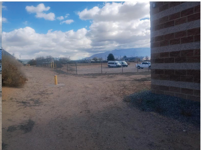
CW-2 settling ponds
