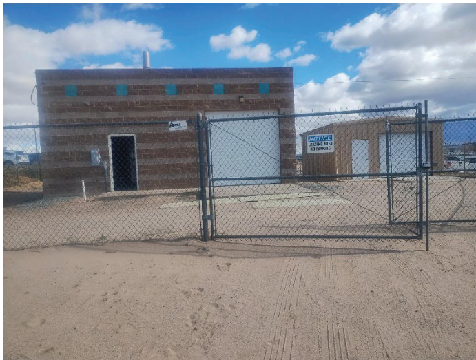
CW-2 Pump house and storage building
