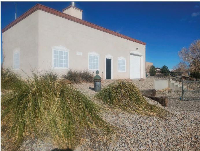
CW-1 wellhead in front of CW-1 pump house
