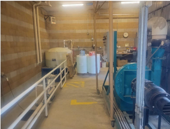
CW-2 Aquamag tank, sump and air stripper
