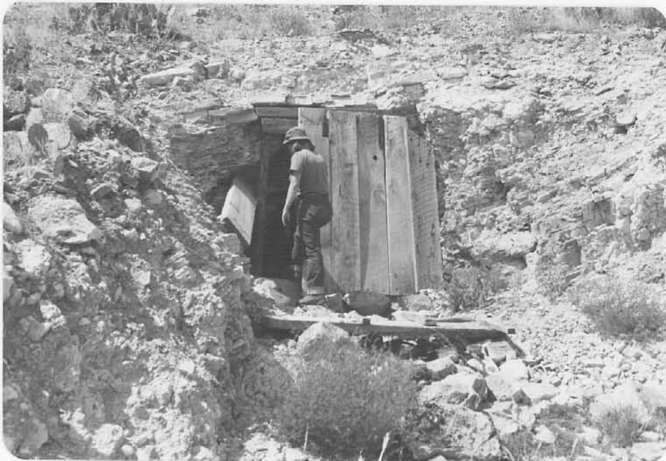
Photo B - first adit, Blue Star.
