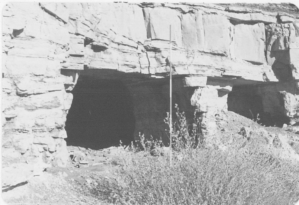
Photo (a) Looking northward into westernmost workings of Rimrock #2 group; entrance to main adit is 6' high; stub adit on right is only 3' deep.
