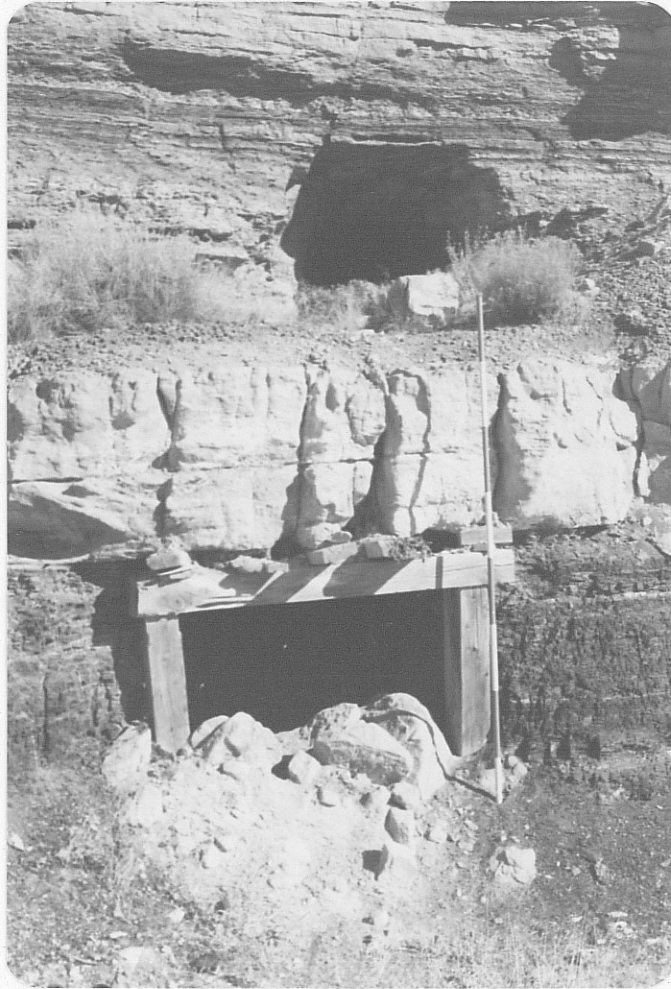
Photo (i) Looking northward into timbered adit in group of eastern sec. 4 workings; note small adit begun above timbered portal.
