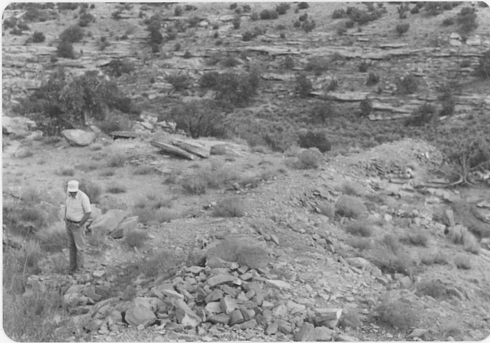
Photo (g) Wheelbarrow run from open cut in foreground to dump in distance.
