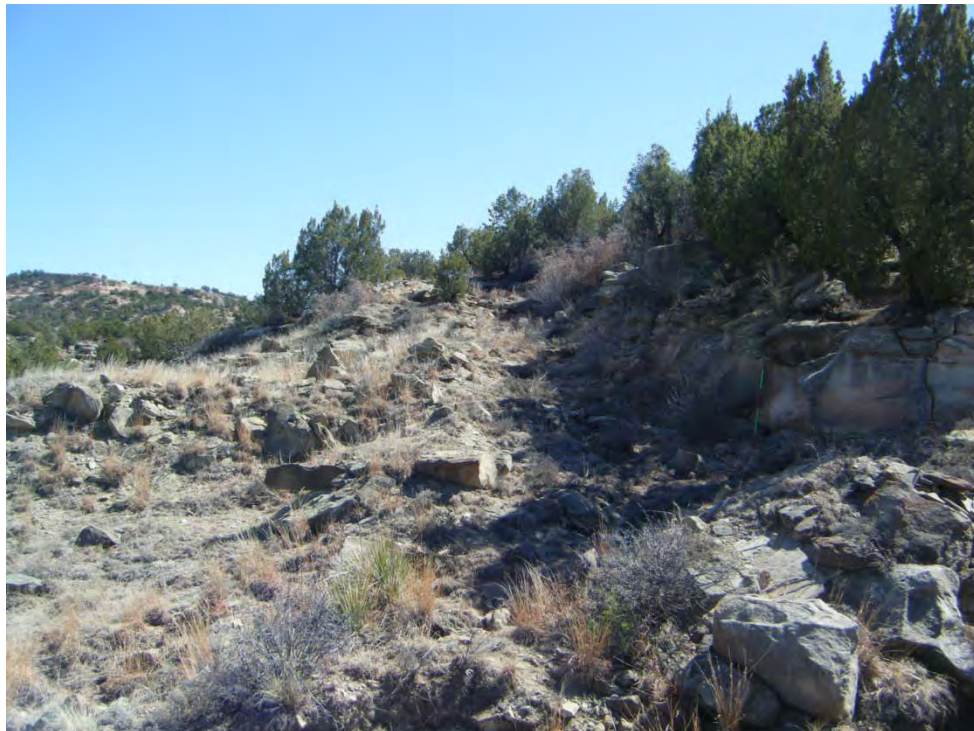
Photo 12-Looking east at PilePly-1 (foreground), PilePly-2 (left background), Rd-2 (center background), and CutPly-1 (right background).
