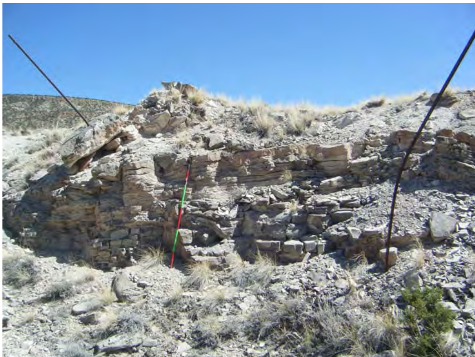
Photo 12-Looking southeast at CutLn-1 (Red Bluff No. 5 claim). Note steel rods in the rock face.
