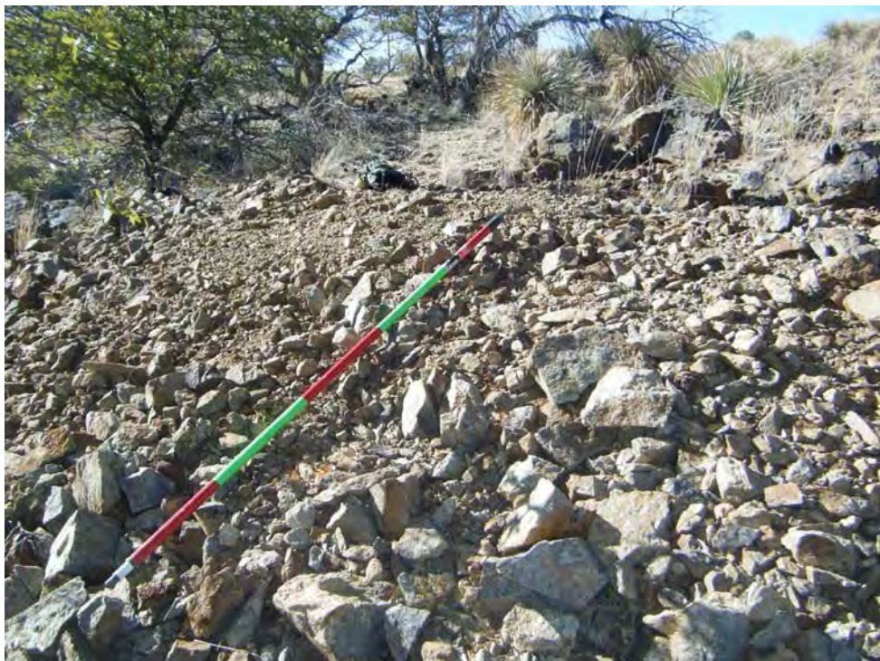
Photo 22-Looking north at PilePly-3, Northern Area.
