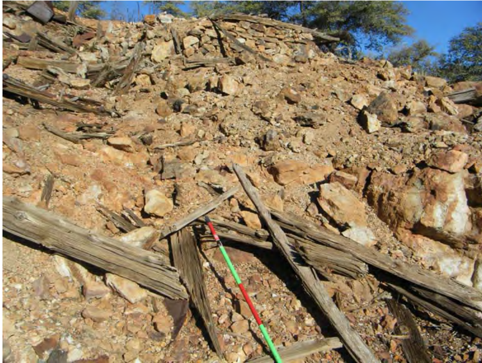
Photo 39- Looking east at collapsed Adit-3, Northern Area.
