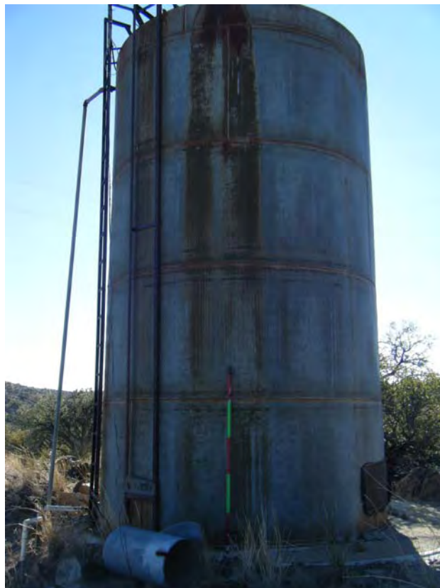
Photo 35-Looking west at the water tank (Tank-1), Northern Area.
