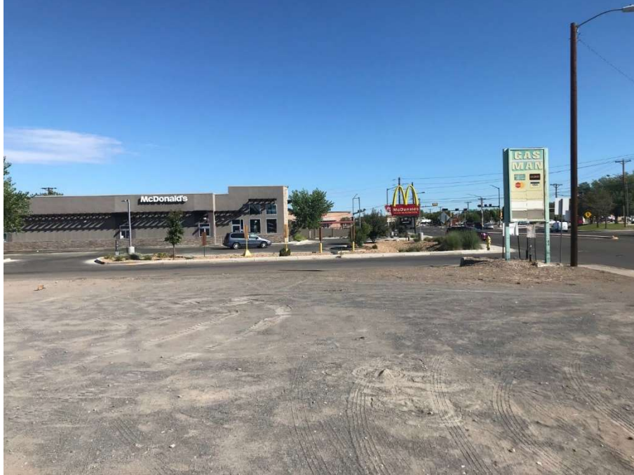
Site After Injection – Facing North
