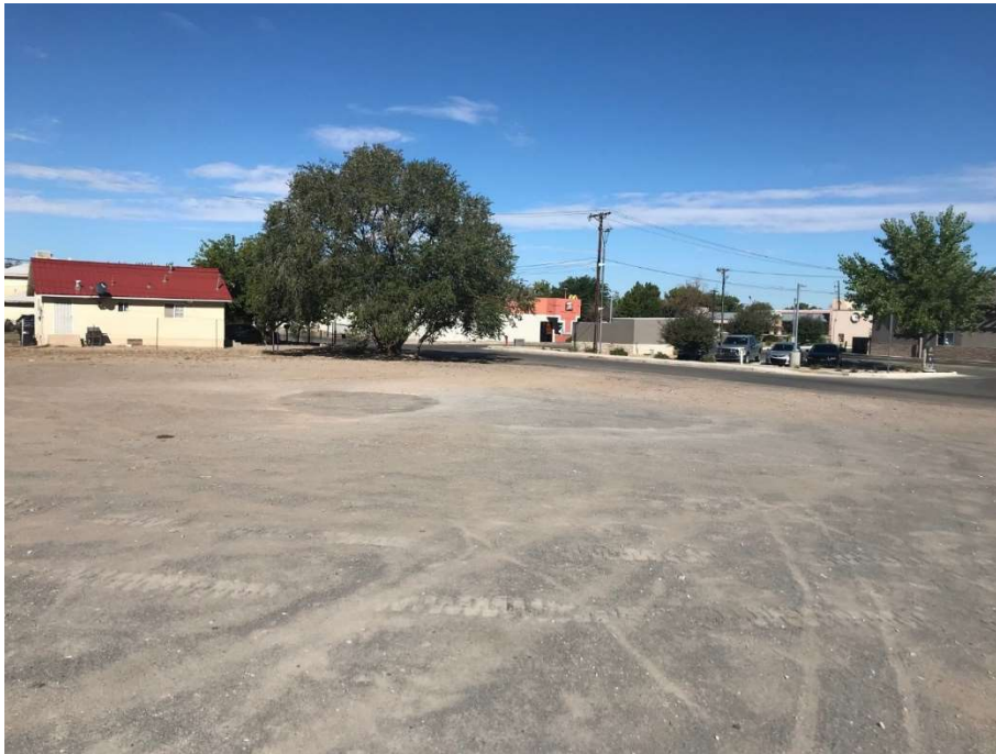
Site After Injection – Facing Northwest
