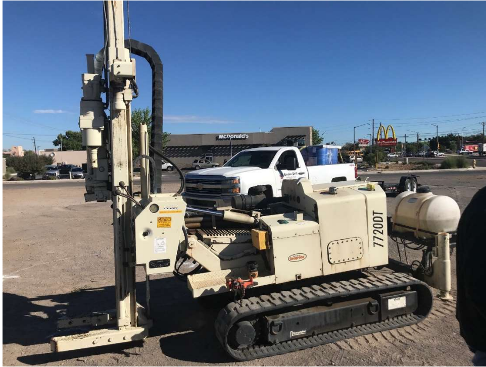
GeoProbe® 7720DT Rid Used to Inject PetroFix®
