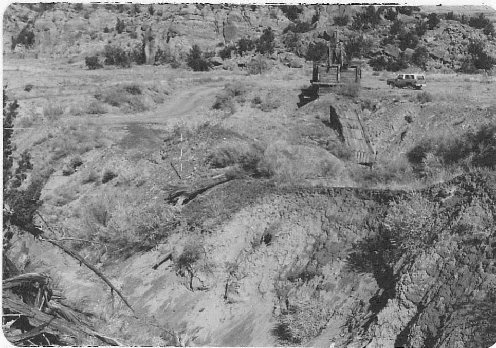
Photo (b) View northward of timbered incline and the headframe and loadout, from drainage line; range pole is on narrow divide between drainage line and caved area over the incline.
