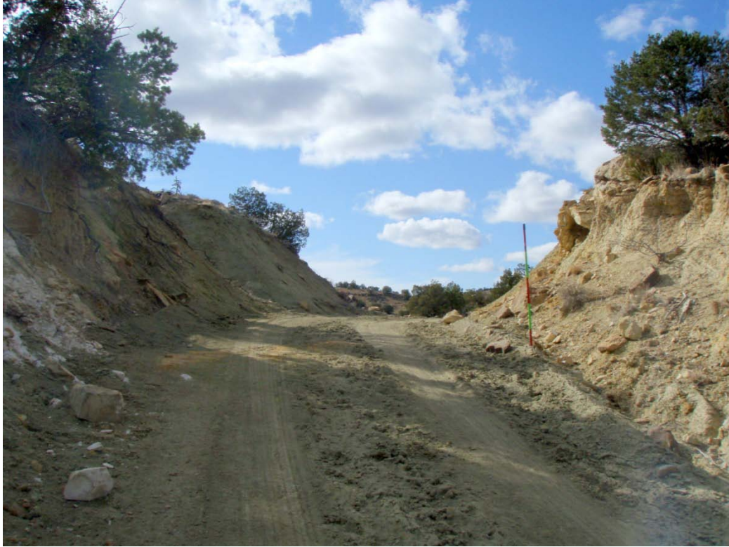
Photo 17-Looking west at CutPly-1. The road Access-1 is visible in the foreground.
