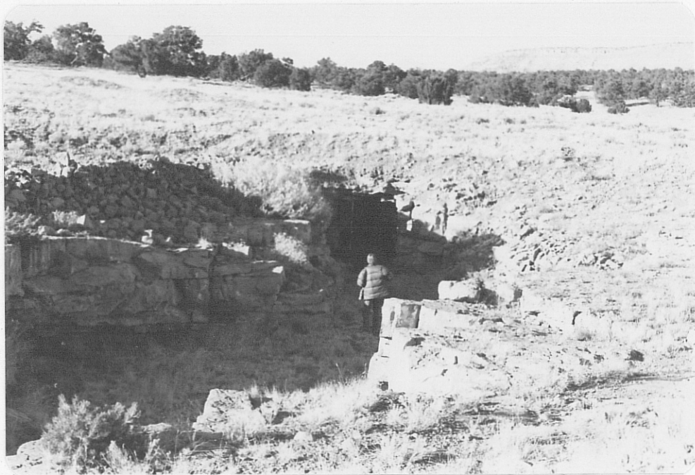
Photo (c) Looking northward at northernmost cut; trench is 110' long with adit at far end.
