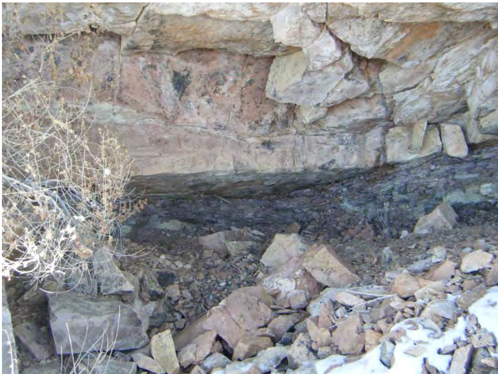
Photo 19 – Adit-1, looking east into slope wall.
