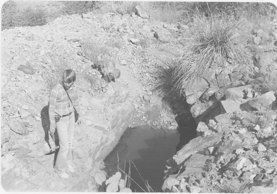
Photo (a) Looking westward at water filled Eugenie shaft; collar dimensions about 4' x 8'.
