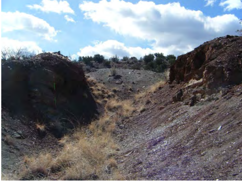
Photo 3-Closer view of CutLn-1 in the foreground and PilePly-1 in the background, looking southeast.
