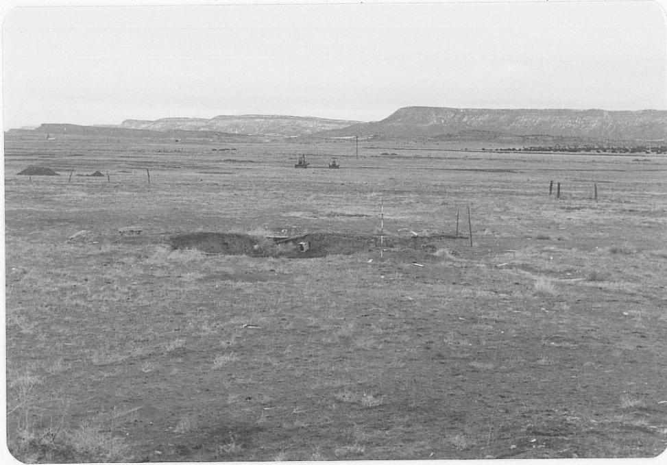
Photo (a) Looking northwest at caved mine shaft site, Rialto Mine; note range pole (center) for scale.
