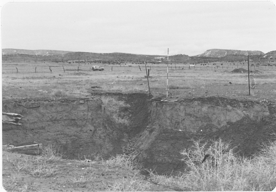
Photo (b) Looking north into caved mine shaft.
