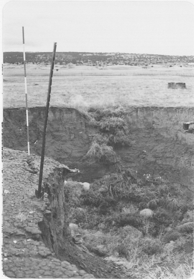
Photo (c) Close-up of caved shaft showing accumulation of tumbleweed at bottom.
