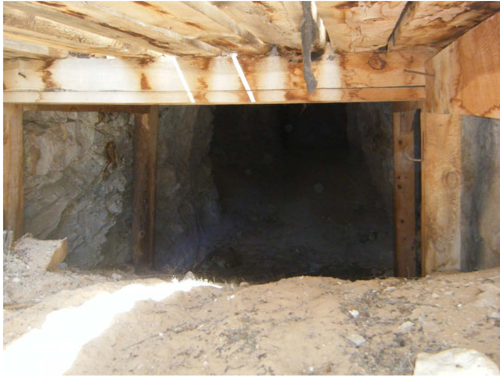
Photo 23-Looking west into Adit-1.
