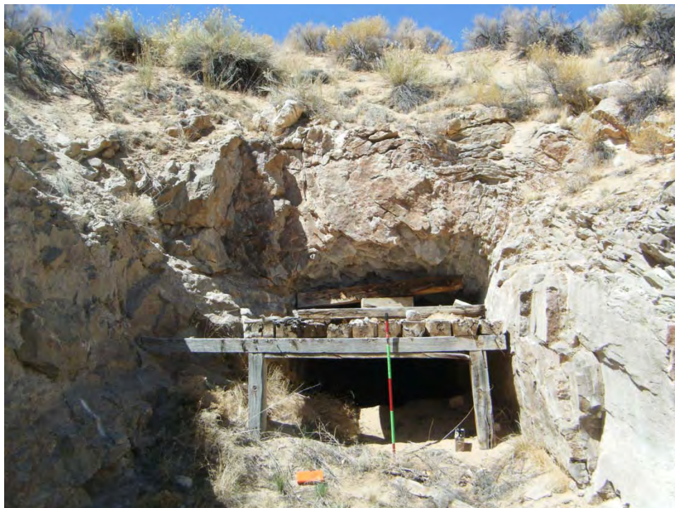
Photo 24-Looking west at Adit-1 entrance, replicating Anderson photo (j). The adit has filled with several feet of blow sand since Anderson visited the Site.
