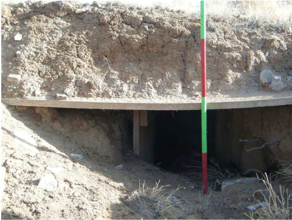
Photo 77-Looking south at StrucPly-2.
