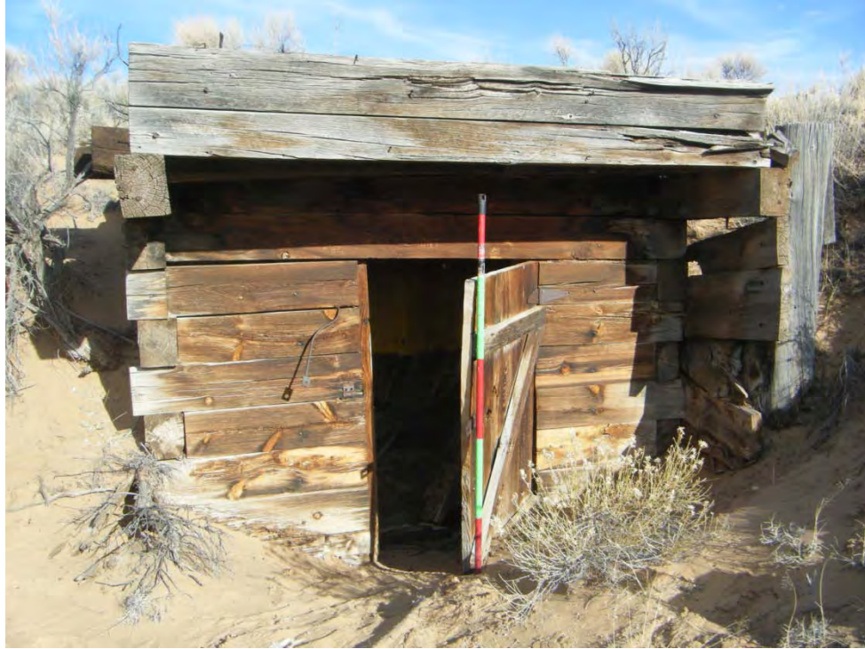
Photo 75-Looking east at StrucPly-1.
