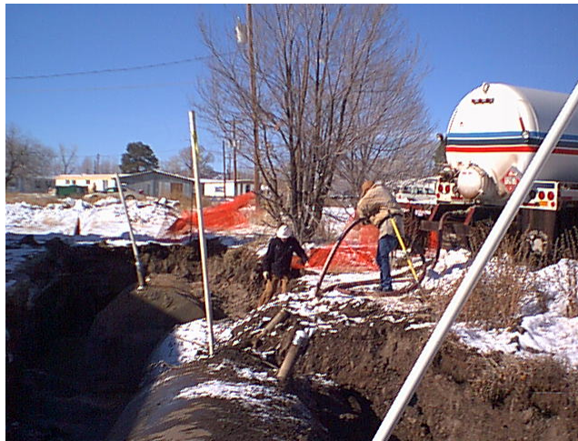
Photo 5: Fluid removal from USTs.
