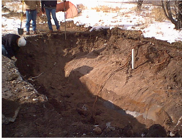
Photo 1: Excavation of UST.
