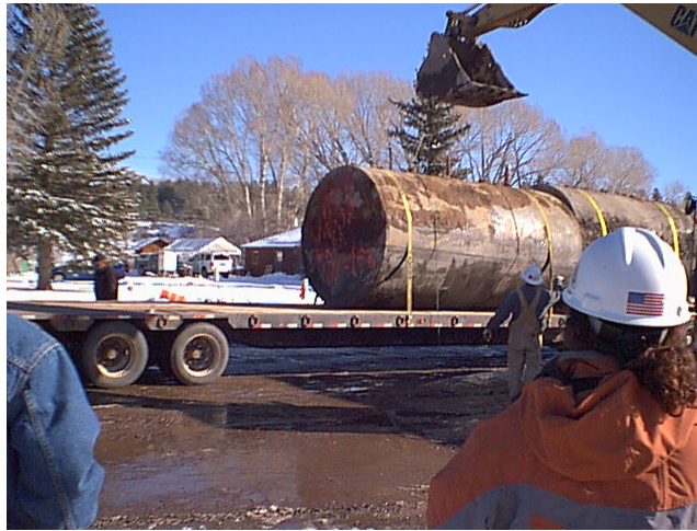
Photo 10: Loading of second UST.
