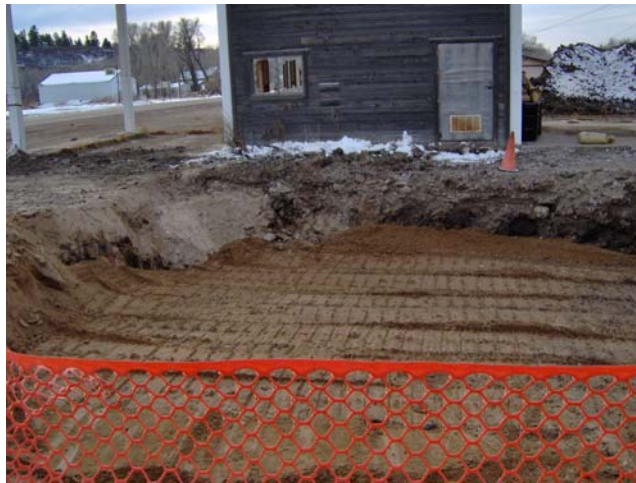
Photo 26: Backfill of excavation area.
