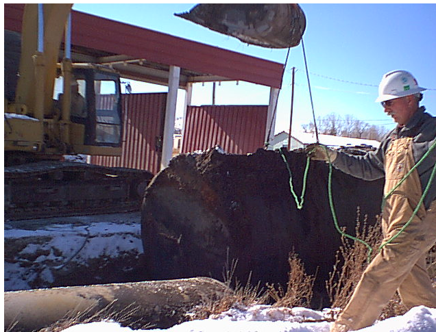
Photo 6: Removal of UST.
