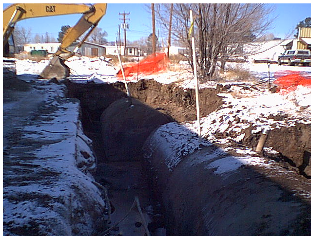
Photo 3: Excavation of USTs.
