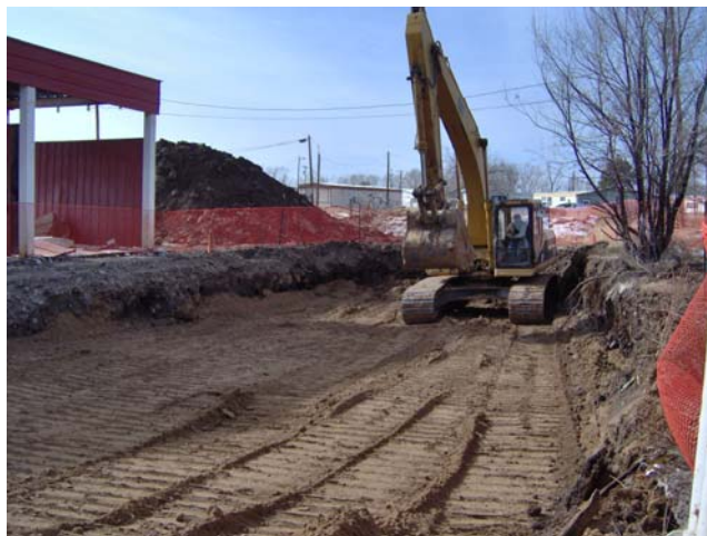
Photo 27: Compaction of excavation area.
