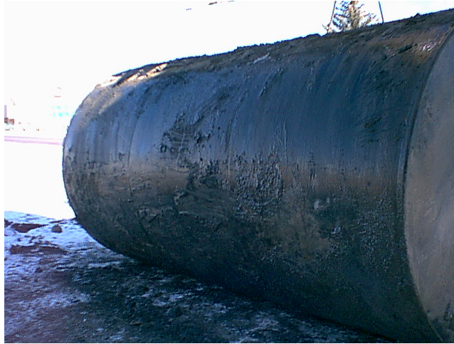
Photo 7: Sheen on bottom of UST.
