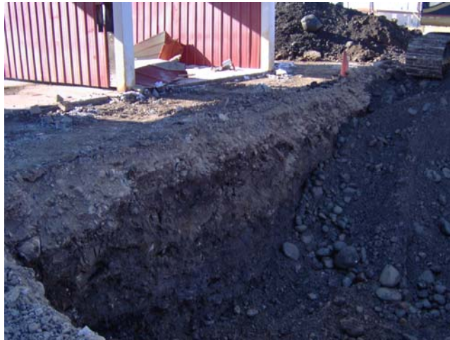
Photo 22: Excavation of second trench.
