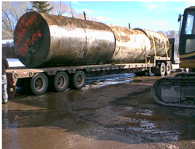
Photo 11: Loading of third UST.
