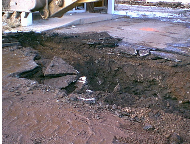
Photo 13: Test pit on southeast side of canopy.
