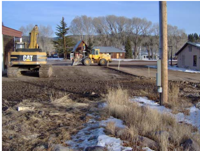
Photo 30: Clean up of site after excavation.
