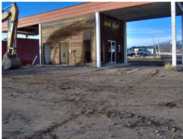
Photo 32: Backfill test pit areas.
