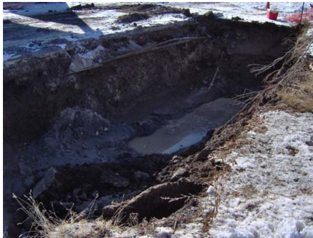
Photo 20: Excavation of UST trench.
