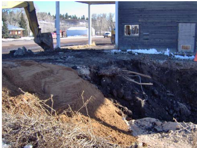
Photo 24: Excavation of second trench.
