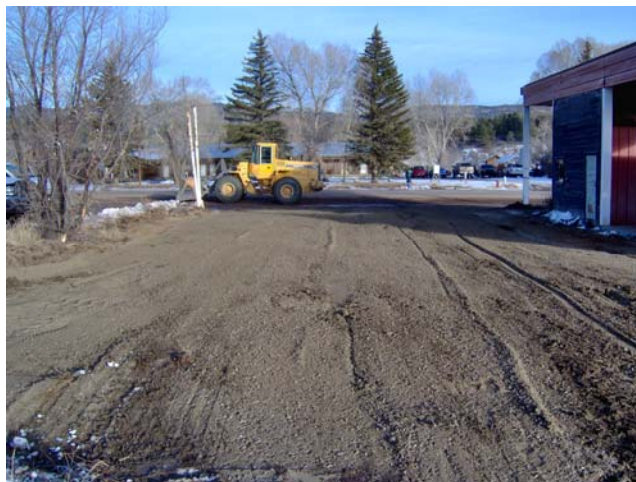
Photo 29: Backfill and final grade of excavation area.
