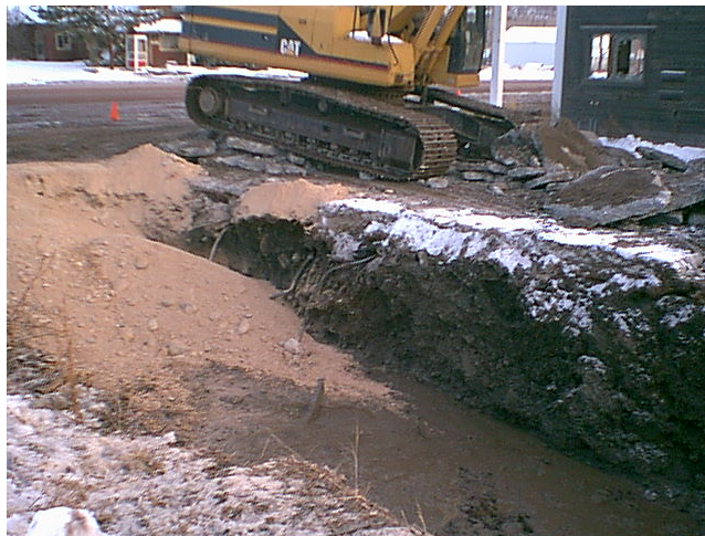
Photo 15: Backfill of tank trench.
