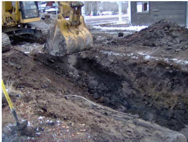
Photo 17: Excavation of UST trench.
