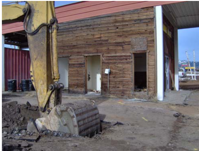
Photo 28: Test pit on south side of car wash.
