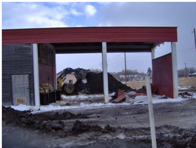
Photo 18: Stock pile of contaminated soils on concrete pad.
