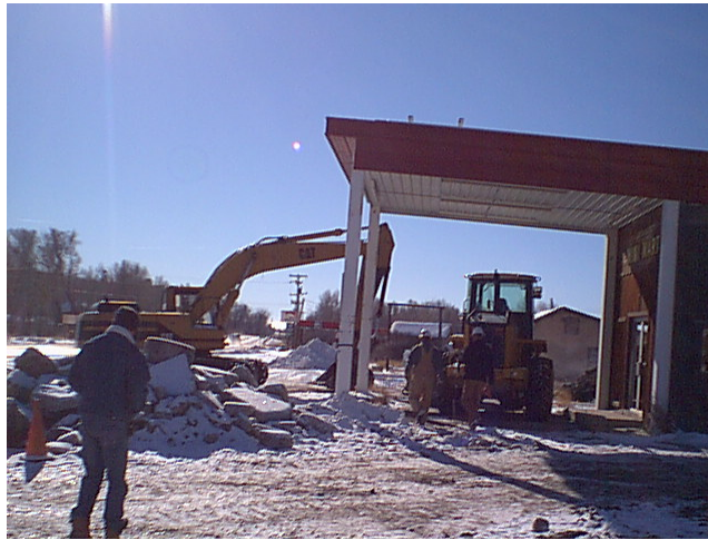
Photo 4: Removal of asphalt and concrete.
