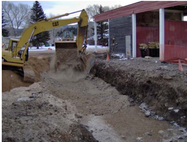
Photo 25: Backfill of second trench.
