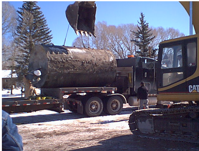
Photo 8: Loading of UST.
