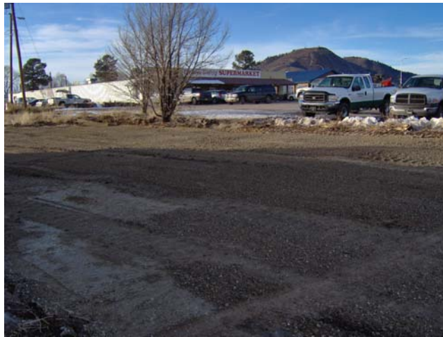
Photo 31: Final grade of excavation area.
