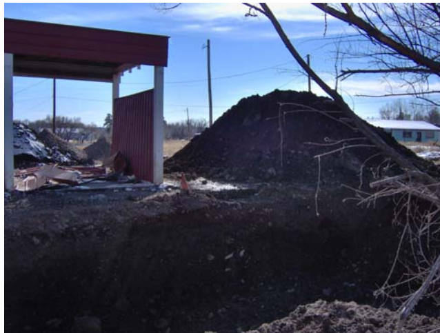
Photo 23: Stock pile of contaminated soils on asphalt pad.
