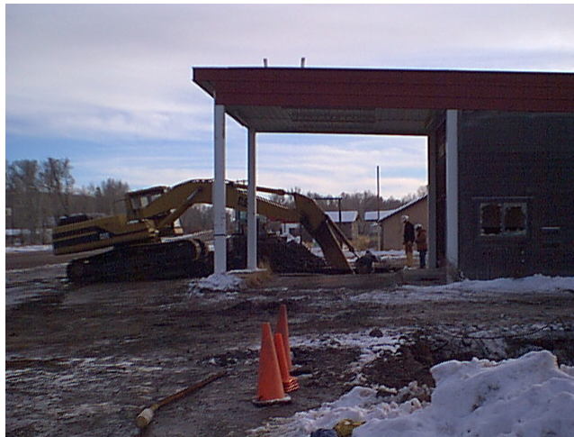
Photo 14: Test pit on southeast side of canopy.
