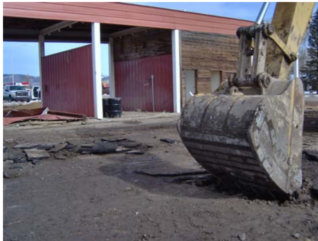
Photo 29: Test pit on south side of car wash.
