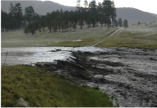
Flooding on Rito de los Indios following the Las Conchas fire of 2011 overtopping the VC09 road crossing with culverts (photo credit: Steve Vrooman)
