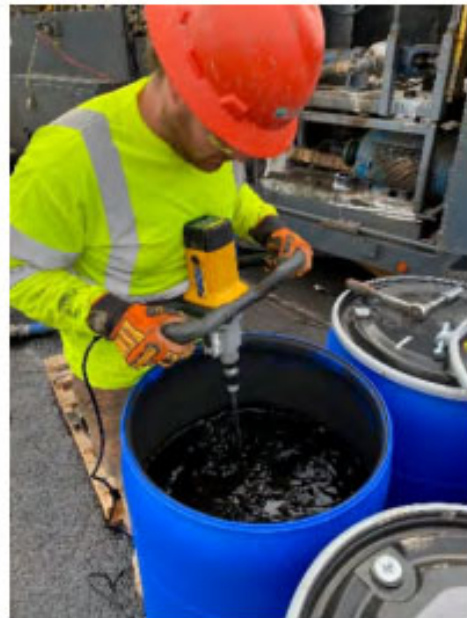
Homogenization of PetroFix using a hand-held paddle mixer
