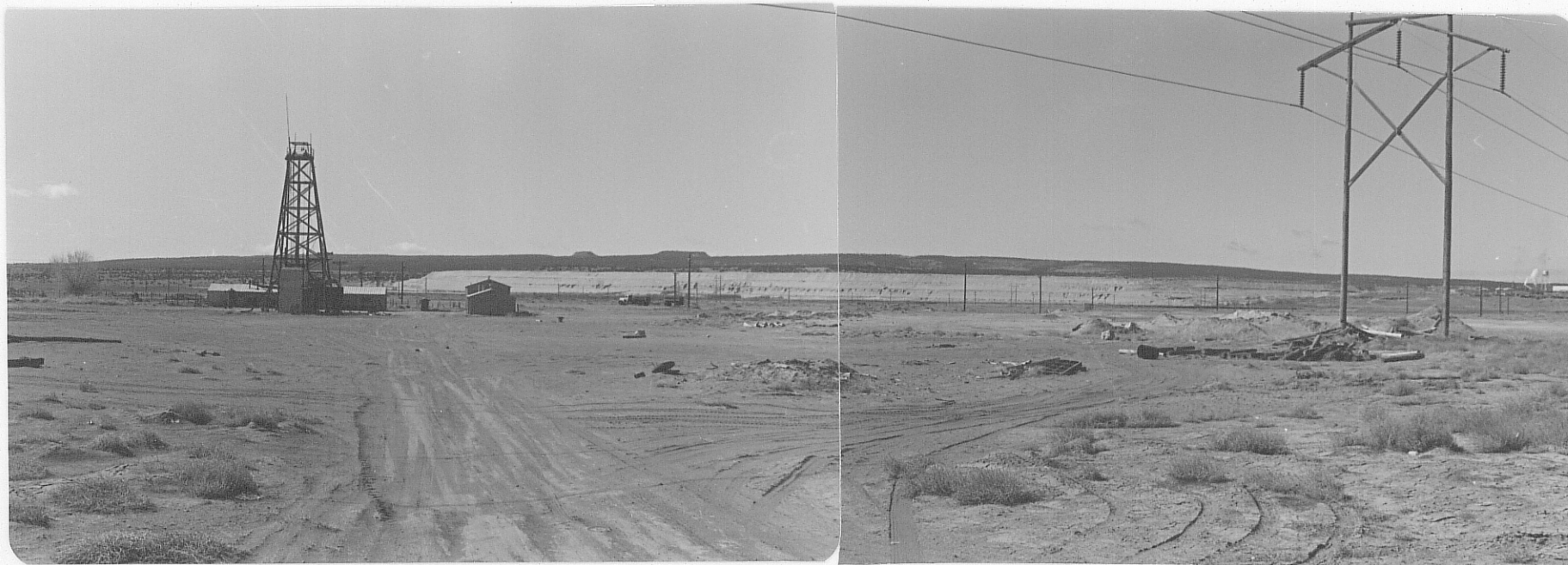
photo (a) Looking southwest at the UN-HP Sec. 32 Mine site and headframe; portion of Kerr McGee Ambrosia uranium mill visible at far right.
