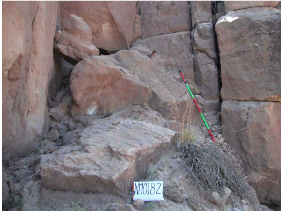
Photo 1-Site location photo, looking south at collapsed Adit-1.
