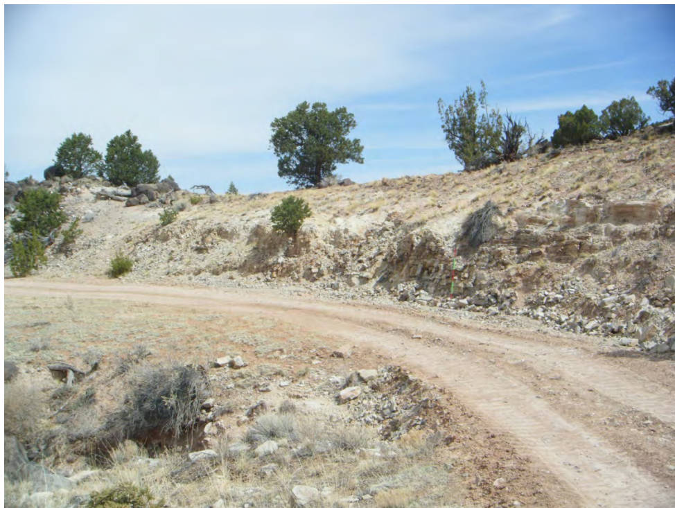
Photo 13-Looking north-northeast at CutPly-5, replicating Anderson Photo (b).
