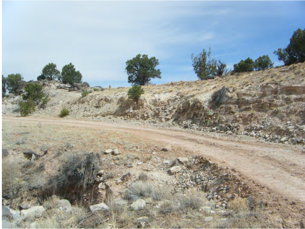
Photo 11-Looking north-northeast at CutPly-5.
