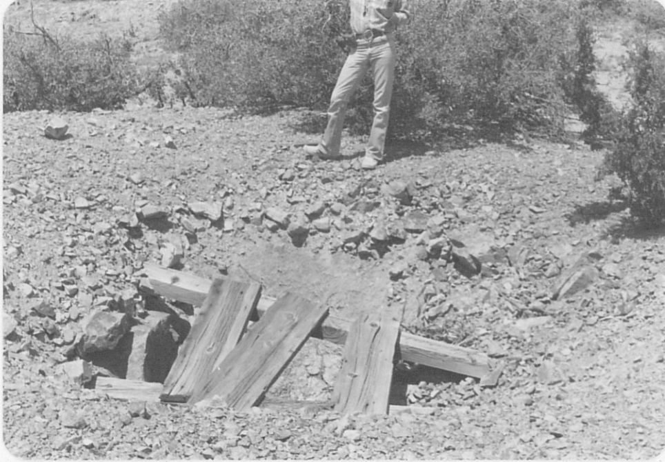
Photo (a) Looking west at Shamrock shaft; collar dimension is 4' x 6'.
