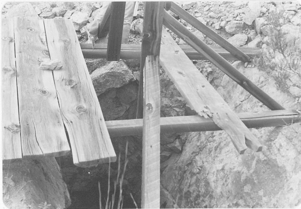
Photo (b) Close up of Alhambra-Bluebelle No. 2 shaft. Depth to water was 10 feet.
