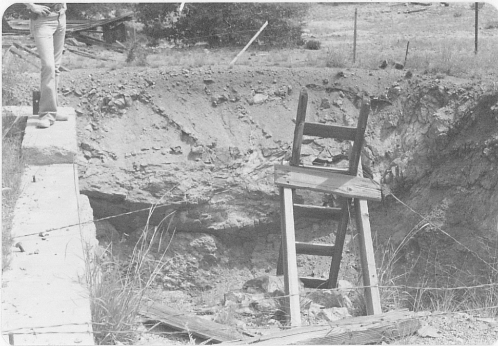
Photo (a) Caved shaft at Floyd Collins Mine.
