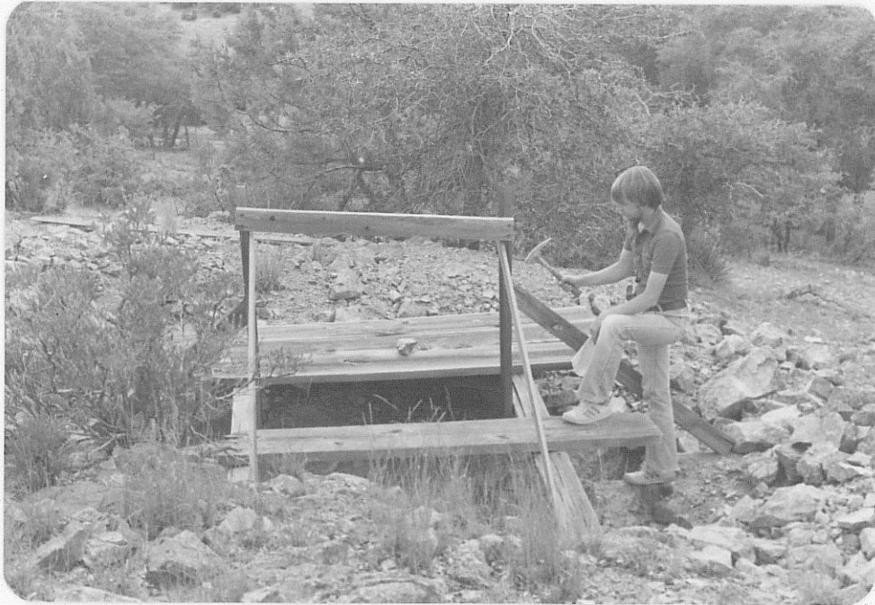
Photo (a) Looking south showing small hoisting platform, underlying shaft, and small tailings pile, at Alhambra-Bluebelle No. 2.
