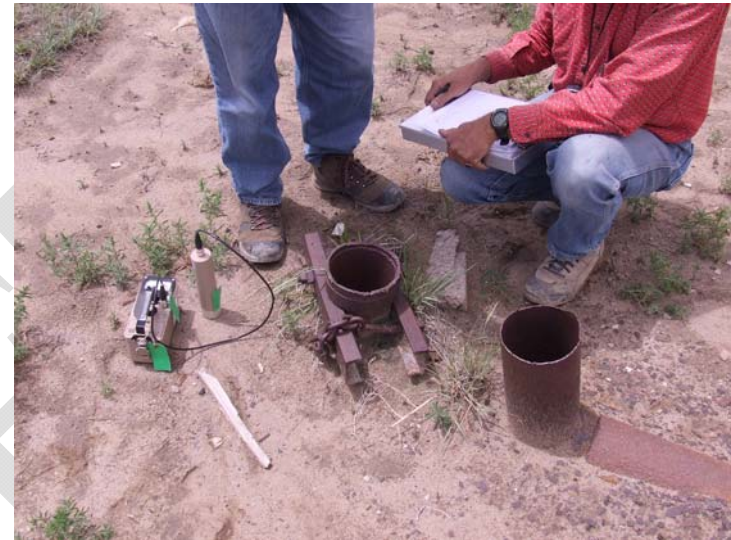
P2: Rusted pipes near shaft; vertical pipe is greater than 100 ft deep
