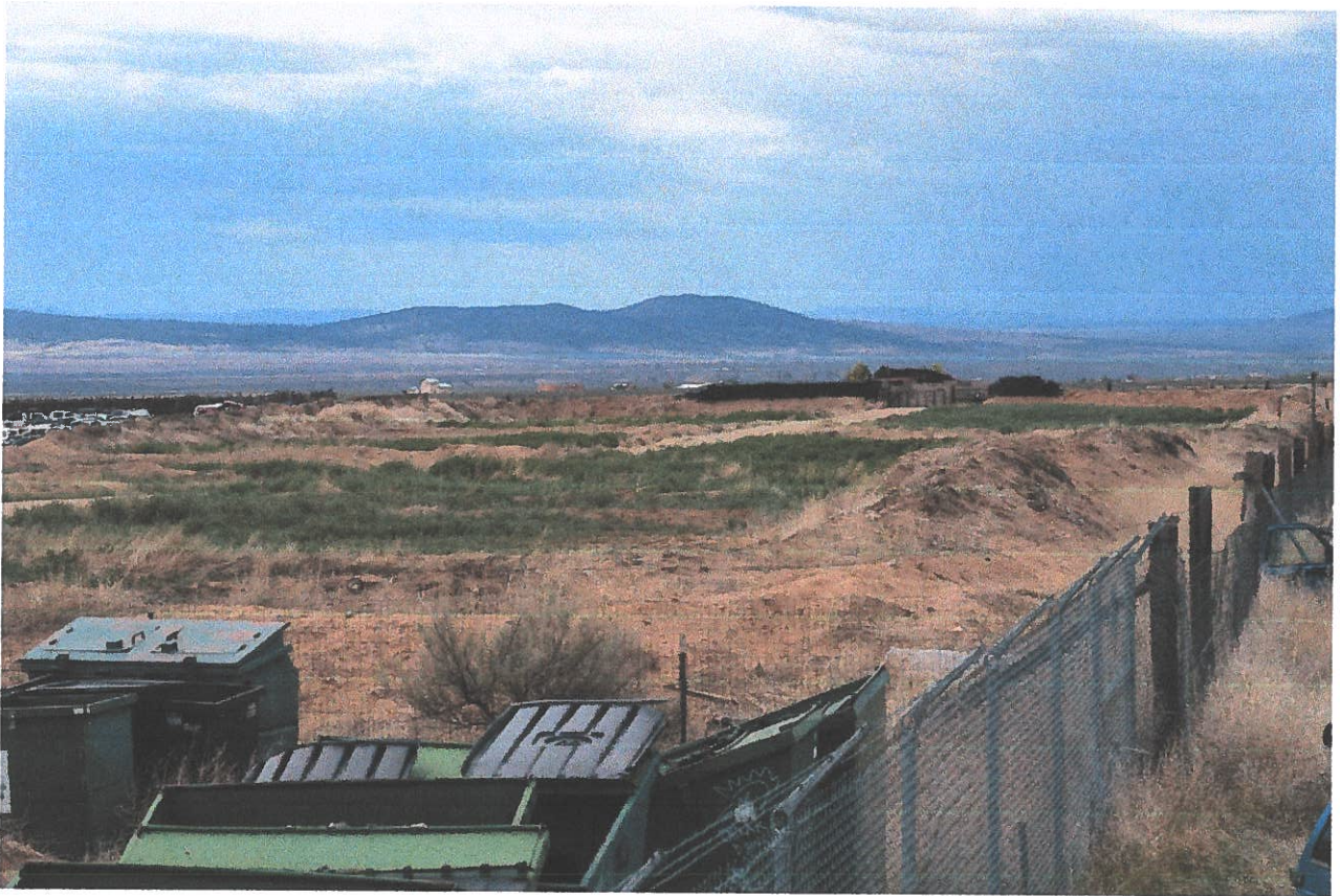
Figure 7. The septic system 7/2018.
