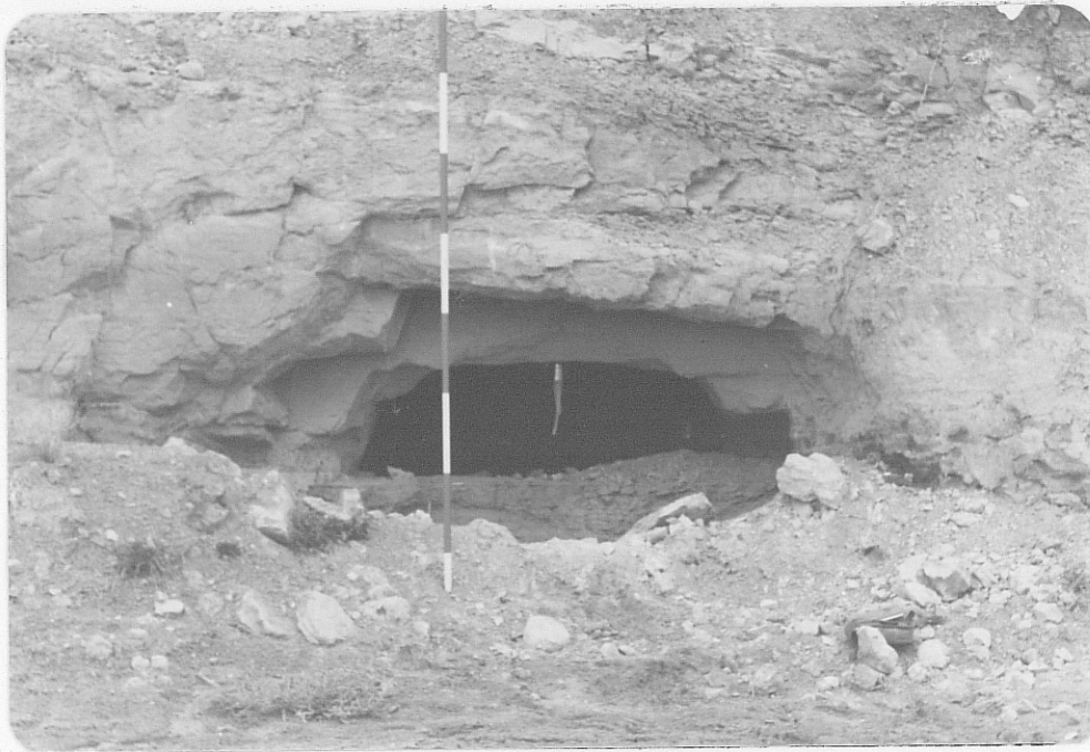
Photo A Looking northward at easternmost workings at Blue Peak; adit is 3\frac{1}{2} ' high, 10' wide, 12' long; (may be only powder magazine but scintillometer read 1700 cps).
