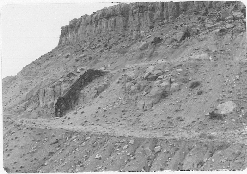
Photo G View westward along south facing escarpment into which Blue Peak adits were driven (upper cut); wooden ore chute extends from adit level down to loadout level, a vertical distance of about 40'.
