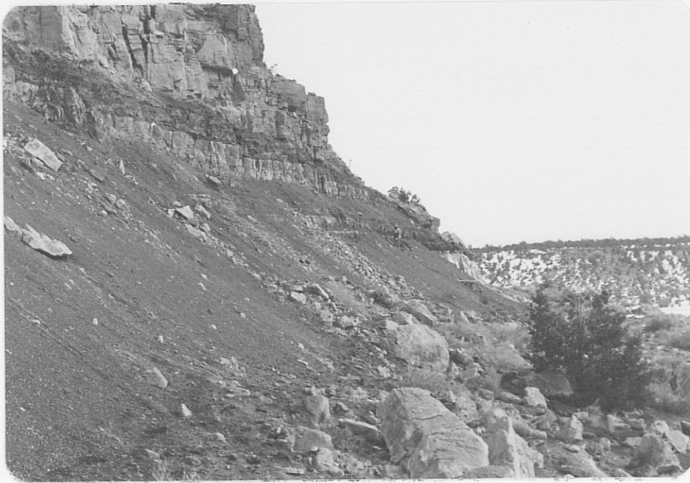
Photo (a) Looking eastward along bench cut at sec. 35 Strip Mine; most of face is natural exposure now made somewhat unstable by 25' cut in soft carbonaceous shales. Note person (center) for scale.
