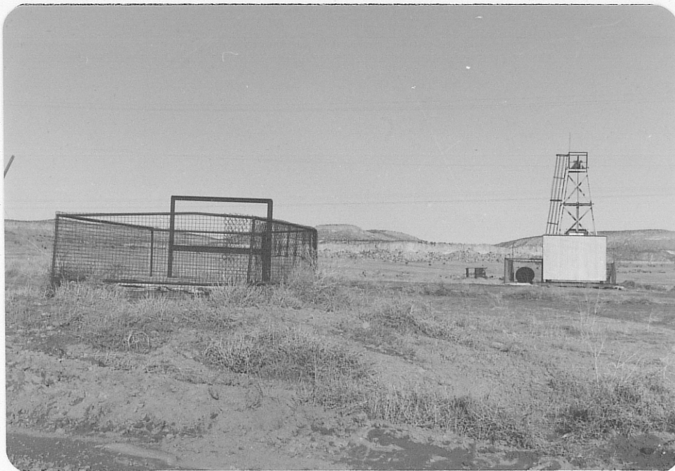
Photo (b) Dysart No. 2 ventillation shaft in foreground, and headframe 150' to east.
