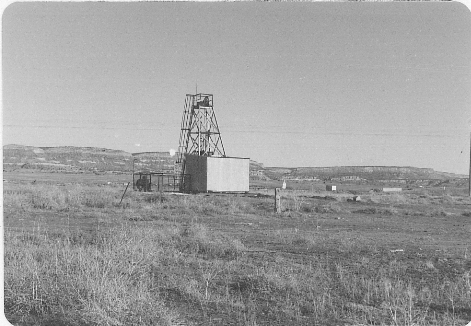
Photo (a) Dysart No. 2 headframe, approximately 30' high; shaft is used as an upcast ventillation shaft by Cobb Nuclear at the Sec. 12 Mine. Cobb equipment is visible in background.
