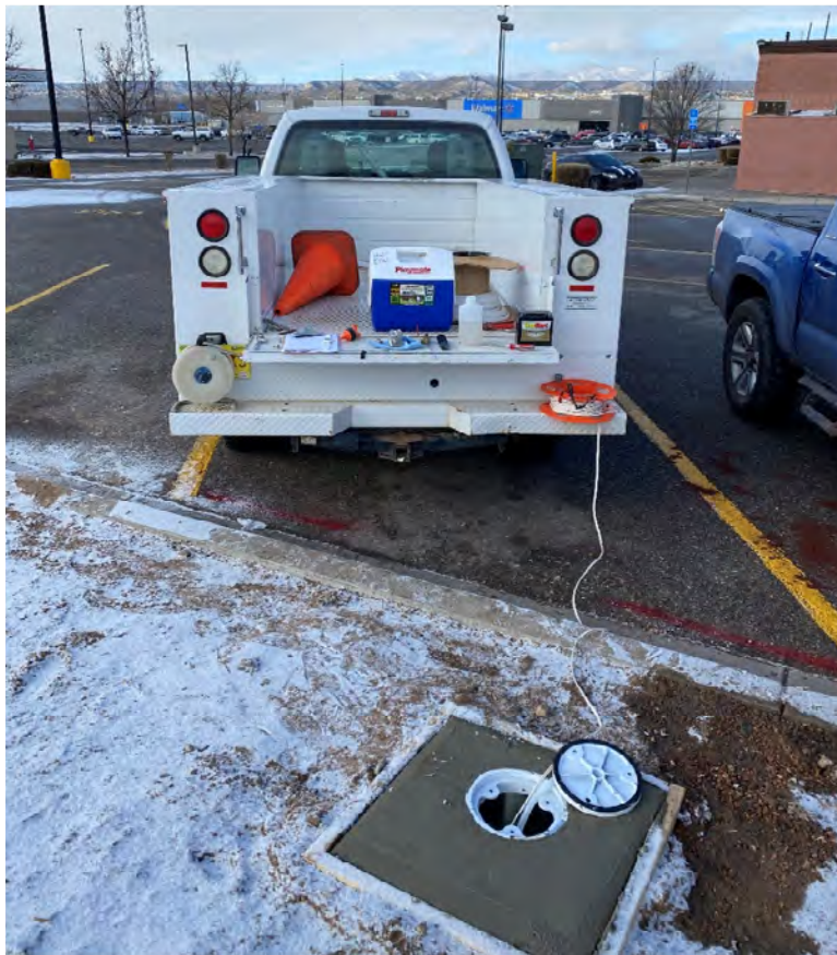
Photo 6 – Developing MW-24 using a submersible DC electric pump.
