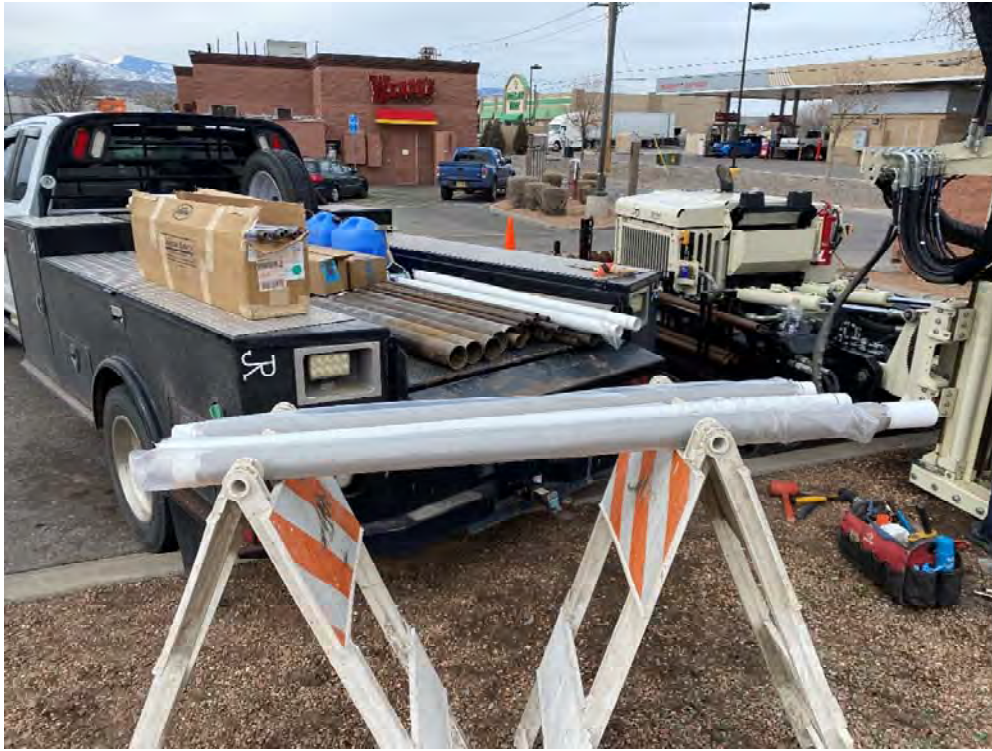
Photo 3 – Prepacked well screen and casing prior to installation in MW-24
