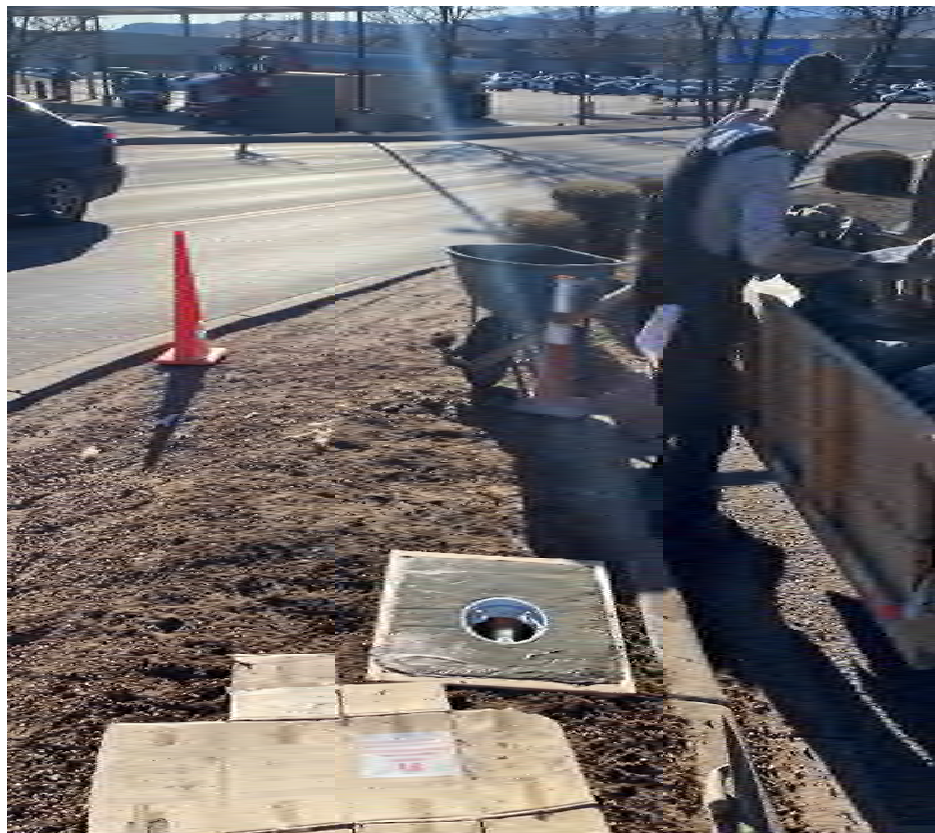
Photo 8 – MW-25 after placing wellhead manway and concrete pad.
