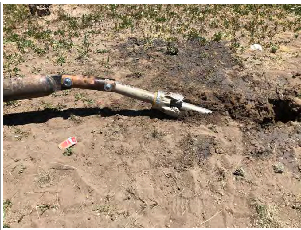
23. Reamer assembly with casing attached for installation
