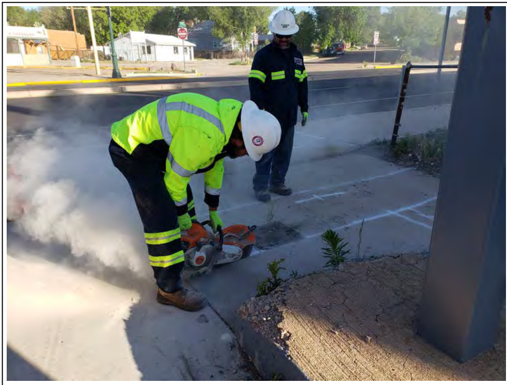
12. Cutting concrete for the exit pit
