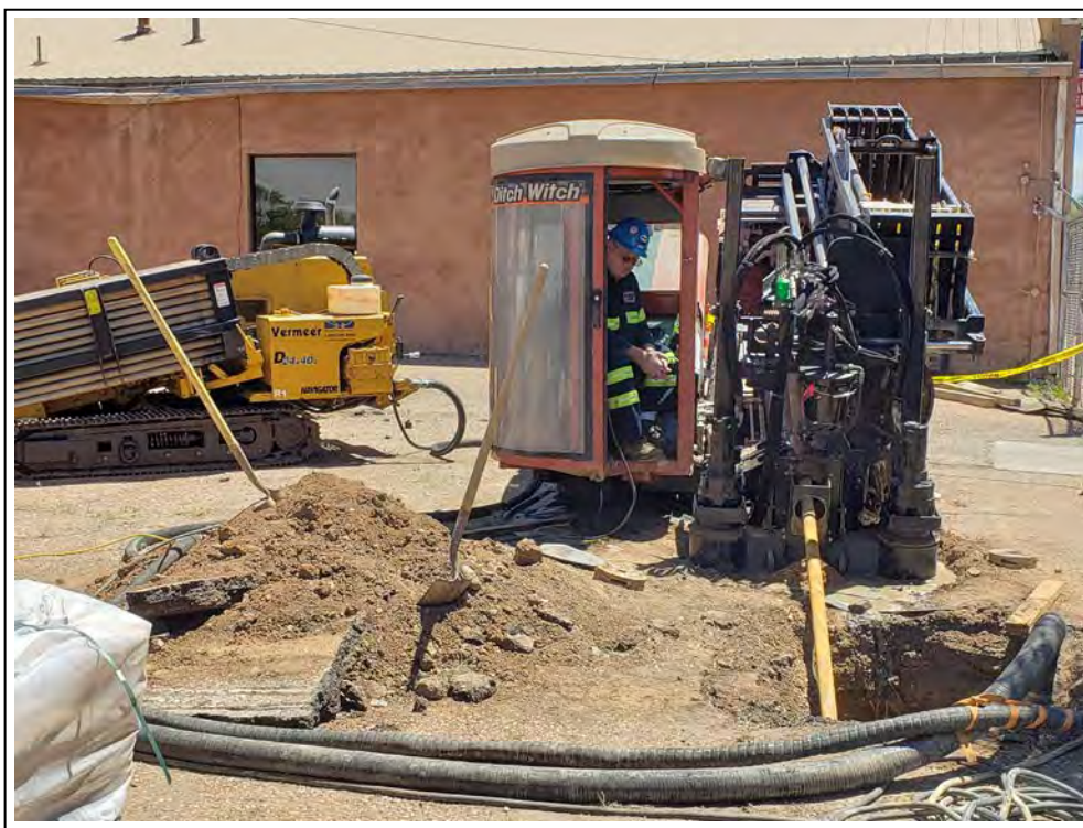
6. Ditch Witch drill rig
