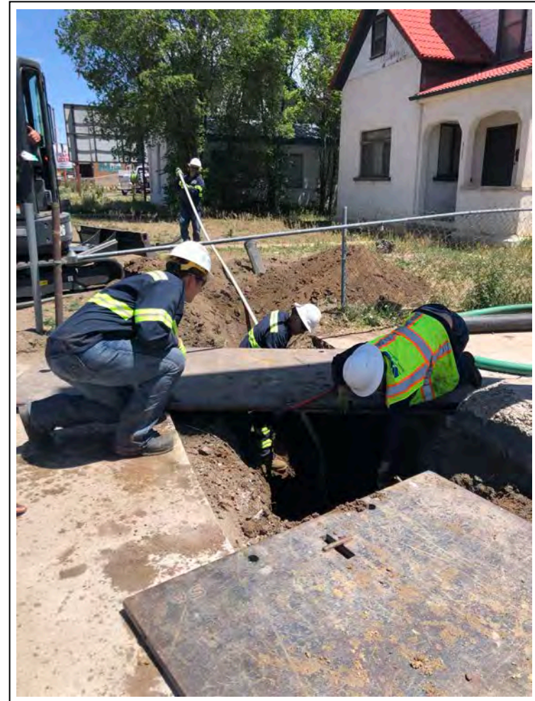
26. Tremmie installed for grouting casing at the exit pit
