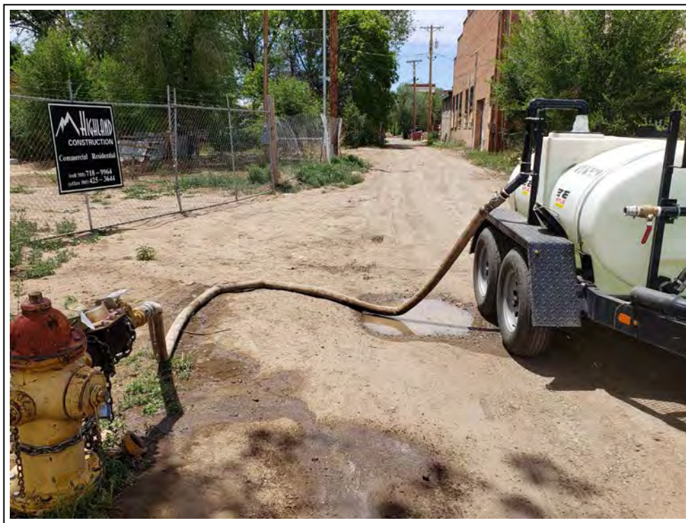
10. Water trailer filling from the fire hydrant
