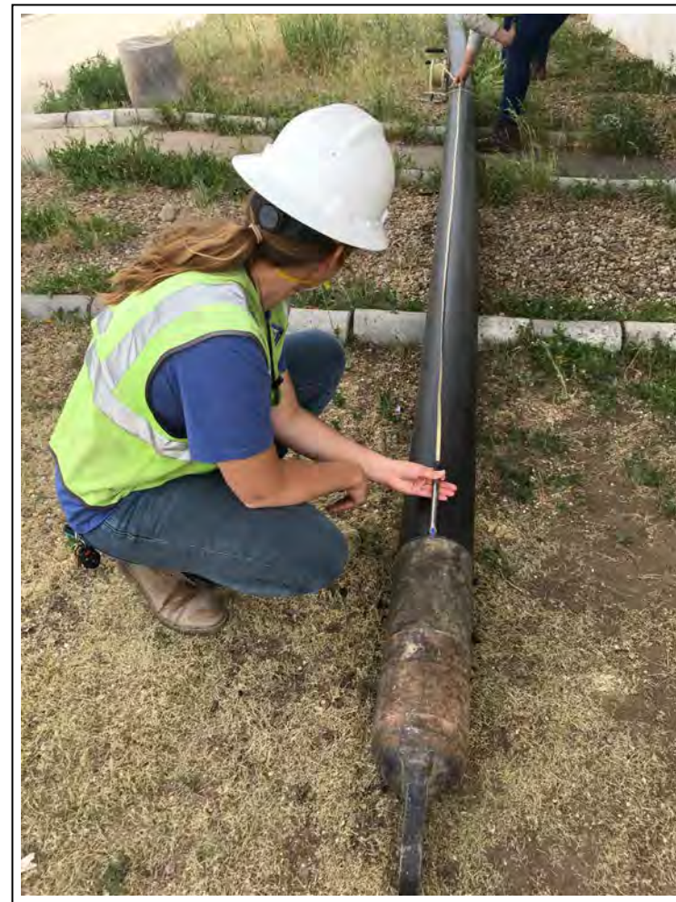
20. 6-inch well casing with the assembly to pull casing into the borehole
