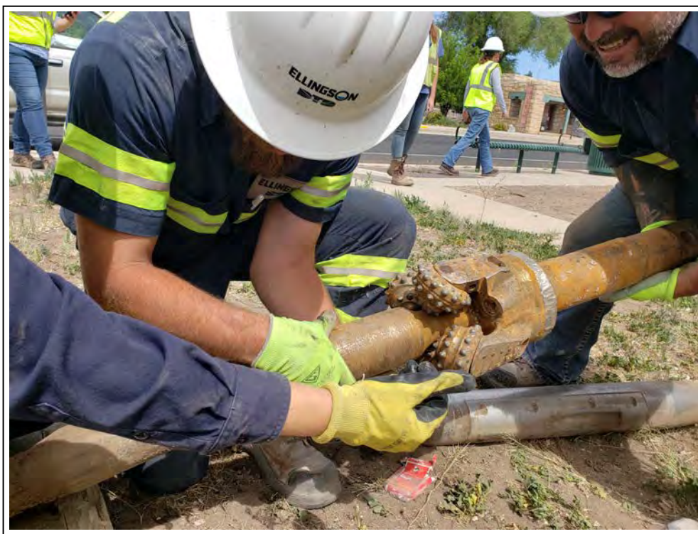
16. Installation of the 8-inch reamer bit assembly
