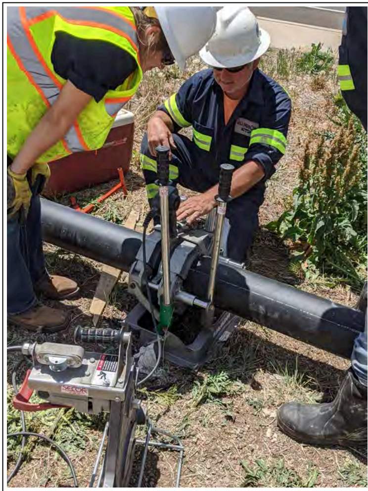
19. Fusing HDPE casing
