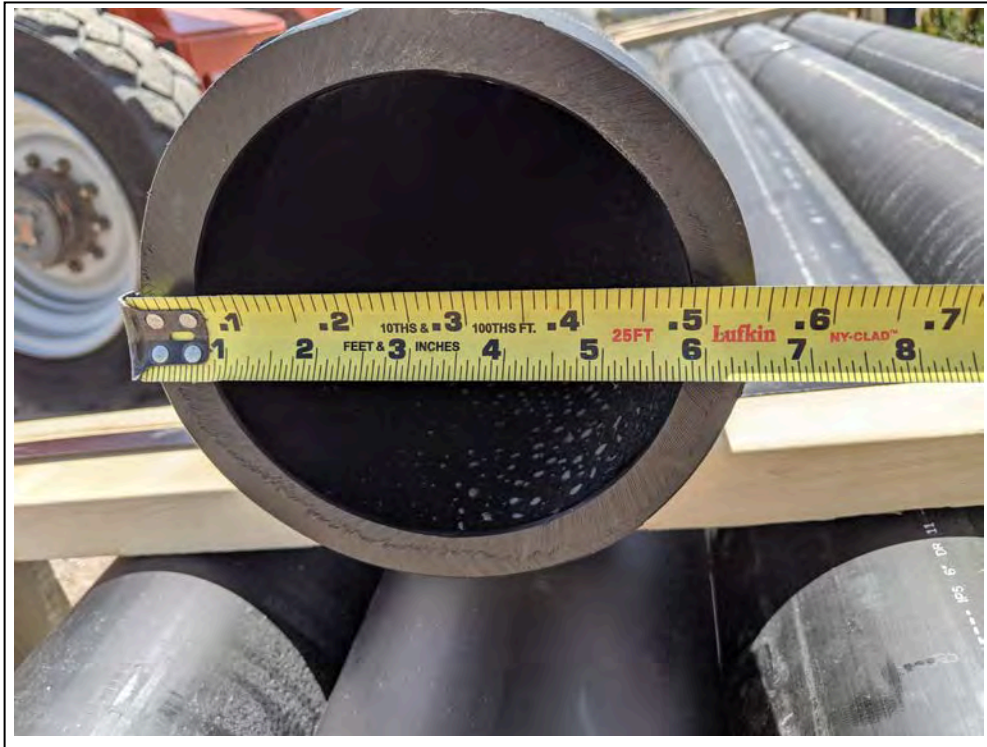
17. 6-inch well casing staged on site
