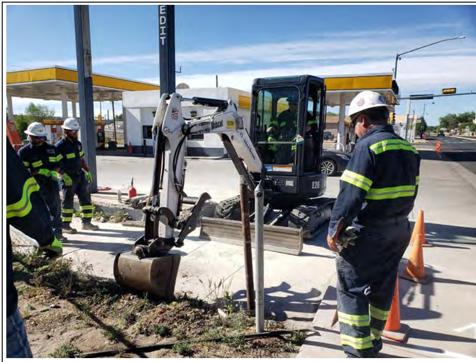
13. Pulling up concrete for the exit pit
