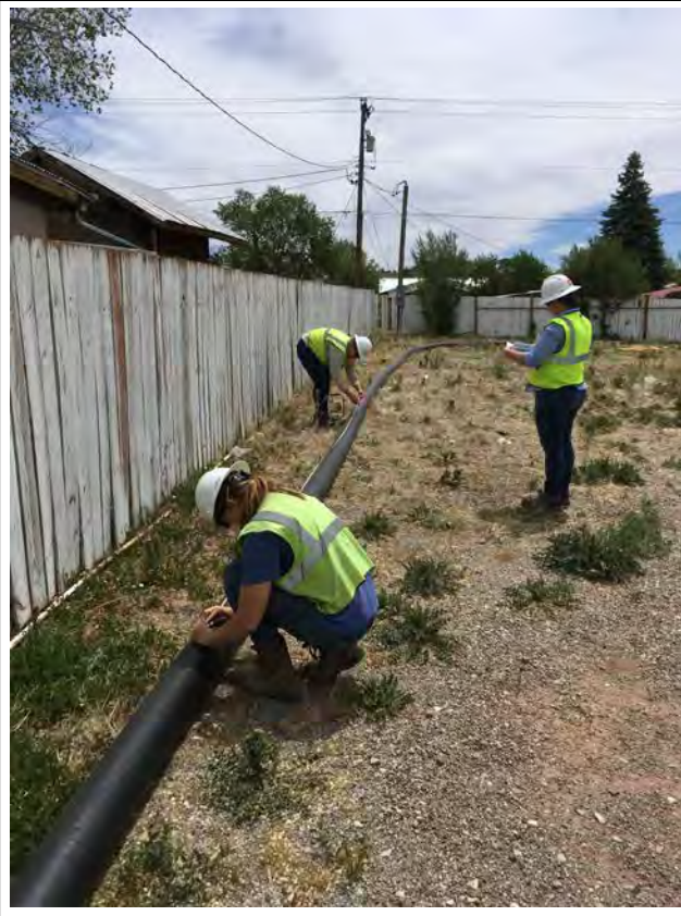
21. Measuring casing materials
