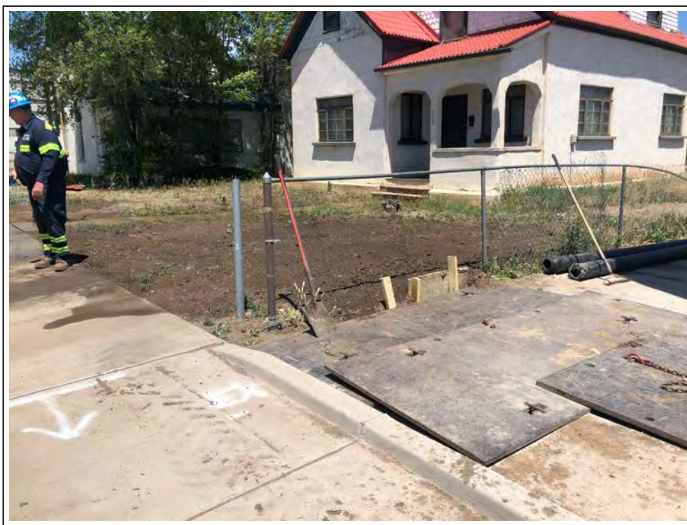
30. Exit pit covered with traffic plates
