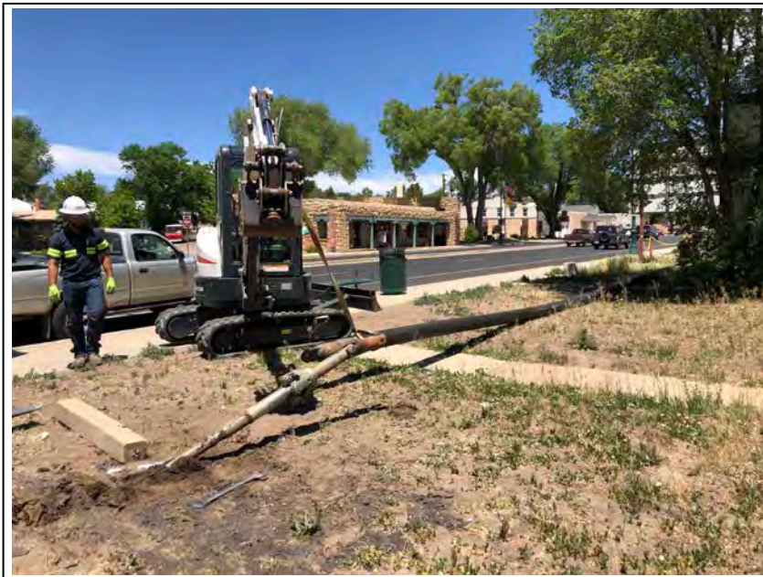
22. Reamer assembly with casing attached for installation
