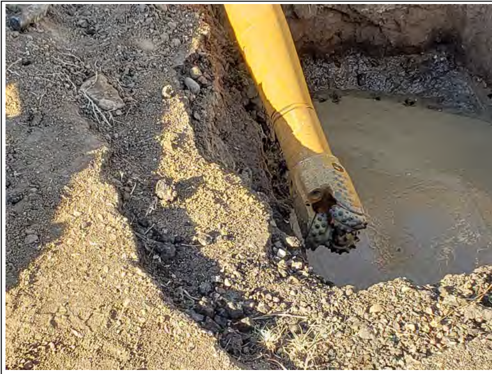
7. Tricone bit and entry pit
