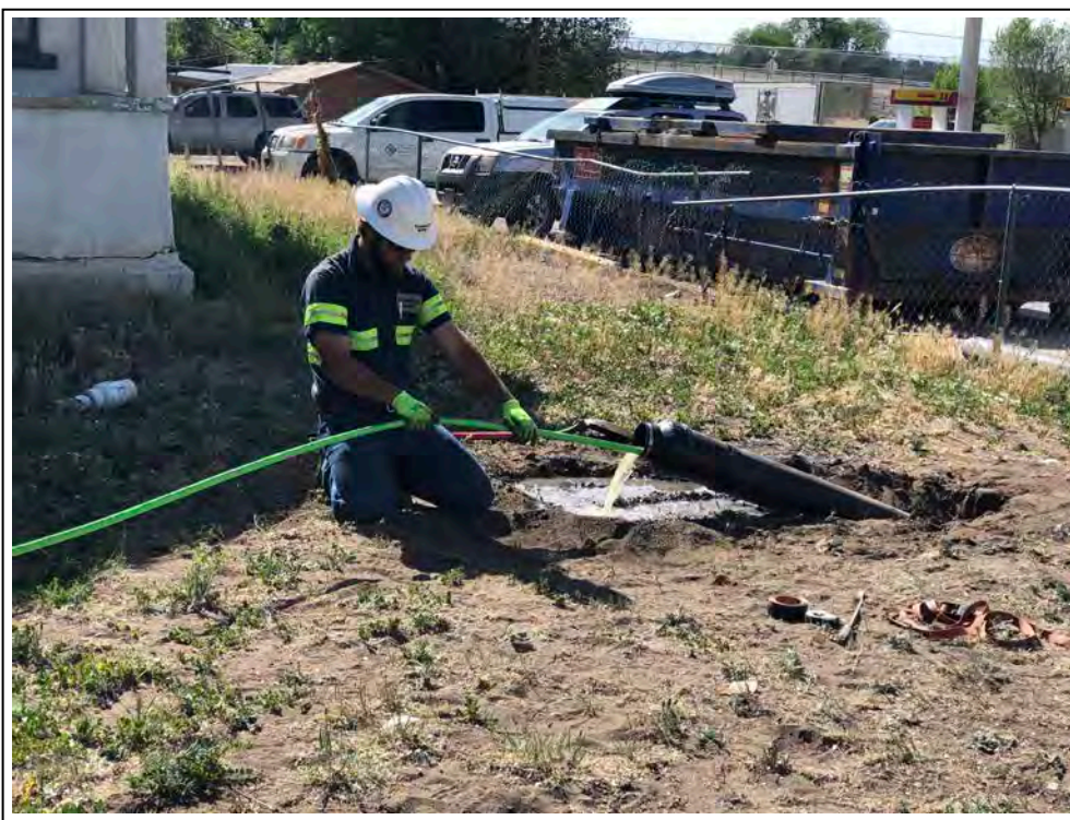
24. Jetting the well screen to develop out drilling fluids
