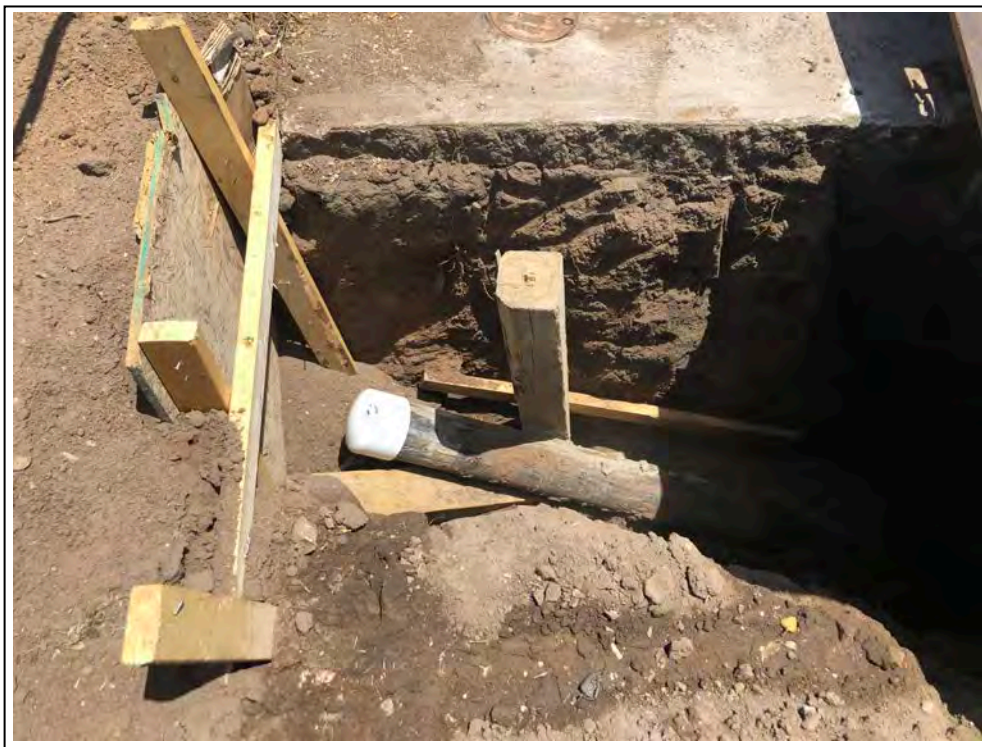
29. Capped casing at the horizontal well exit pit
