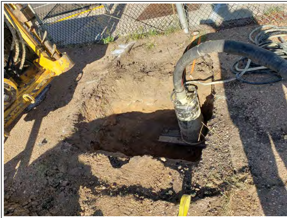
2. Entry pit with pump for mud recycling system
