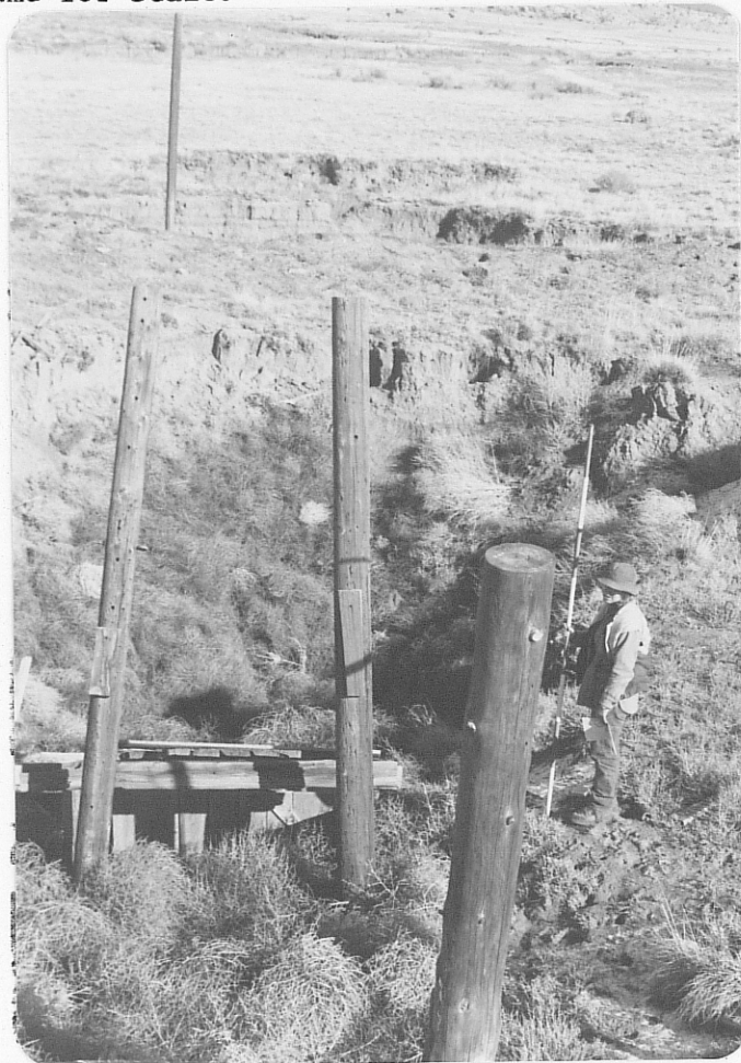
Photo (b) Looking northward from atop headframe down the collapsed decline. Note 3 separate collapse features, the first one being at the portal.
